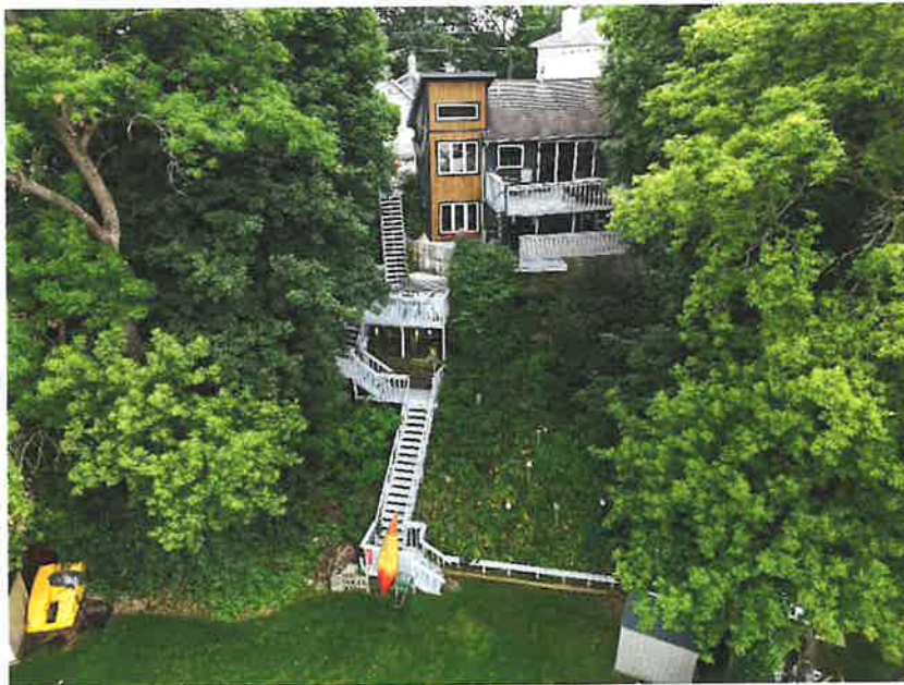
Photo 1 – Existing Residence and Property, Viewing South
