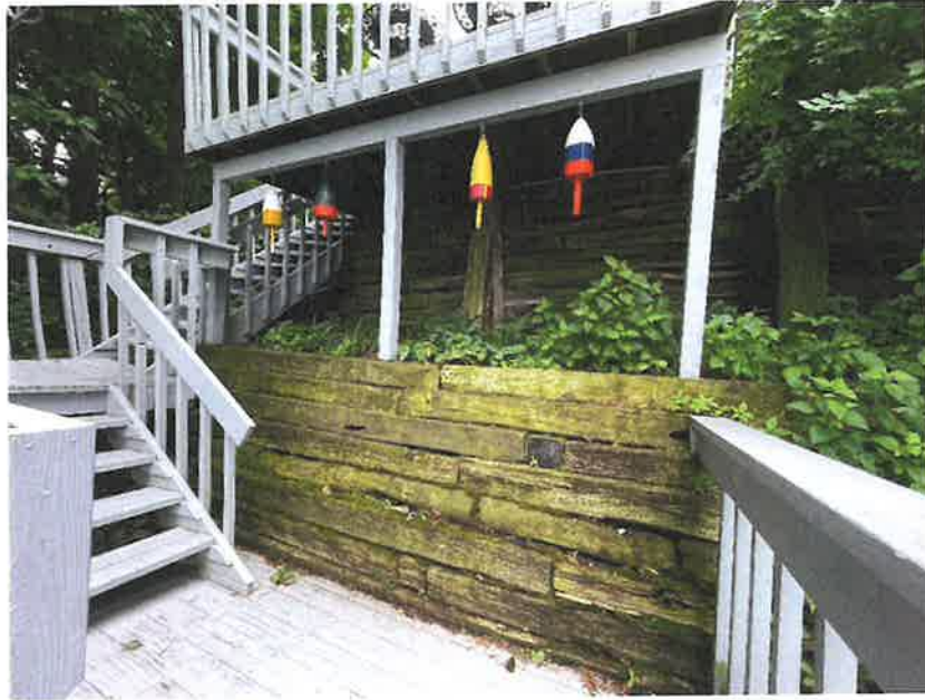
Photo 4 – Portion of Retaining Wall 1, Looking North from Wood Stairs (Retaining Wall 2 Visible in Beyond)
