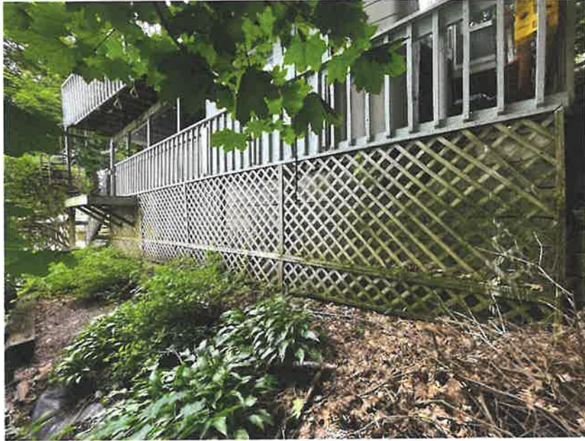
Photo 16 – Portion of Retaining Wall 3 below Patio, Viewing Southeast
