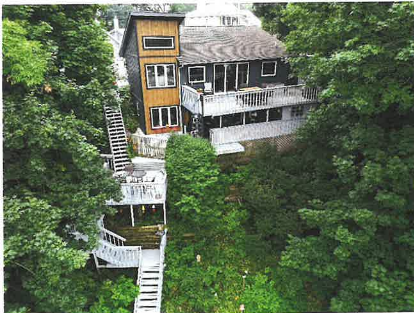
Photo 3 – Existing Residence and Property Enlarged, Viewing South (August 6, 2026)
