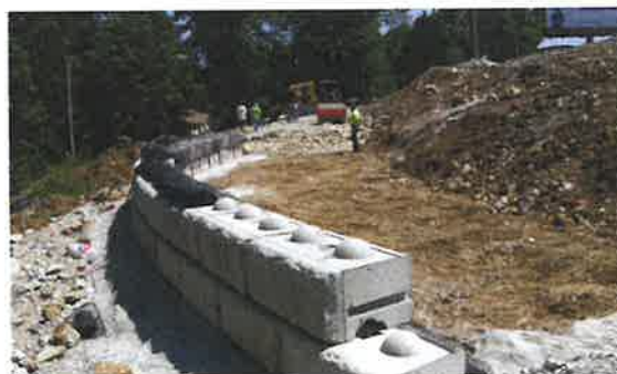
Figure 5 – Conceptual Example Photo of Retaining Wall Installation
