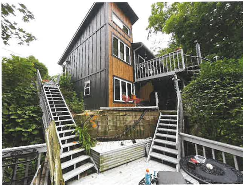
Photo 17 – Portion of Retaining Wall 3 at Curve, Viewing Southwest
