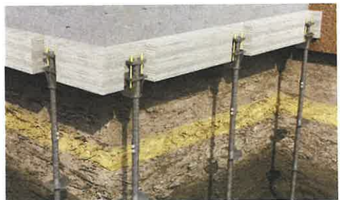
Figure 5 – Conceptual Example Photo of Helical Piers
