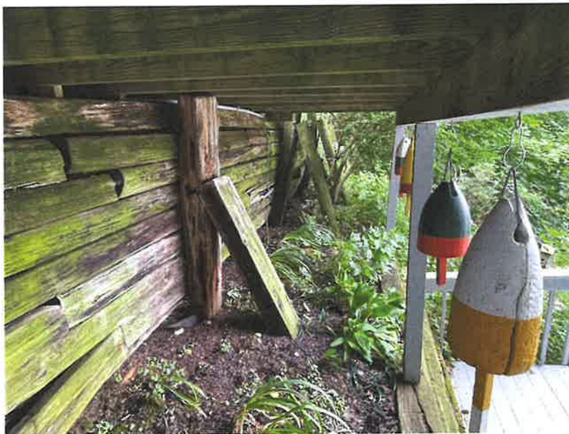
Photo 9 – Retaining Wall 2, Viewing Southwest from below Upper Deck
