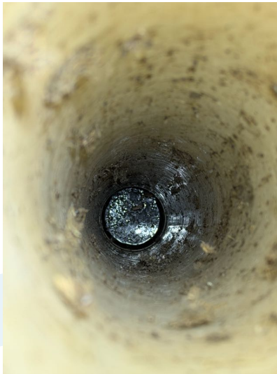
some water observed in one observation port
