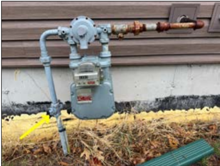
Main gas valve shut off
