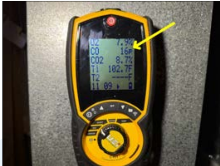
Good combustion levels
