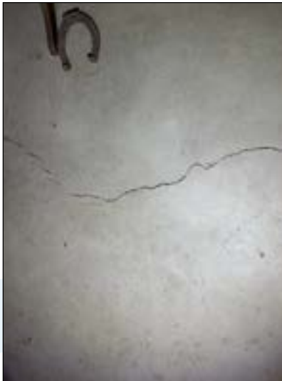
Typical cracking
