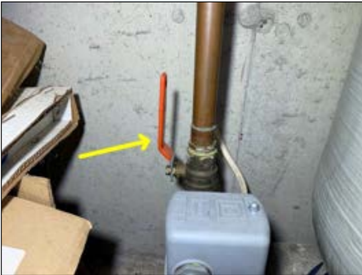
Main water shut off
