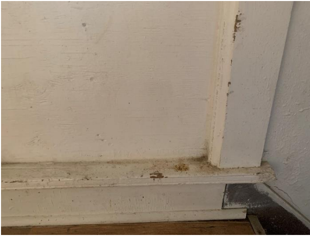
Window Casing (Outer) Back Entry
