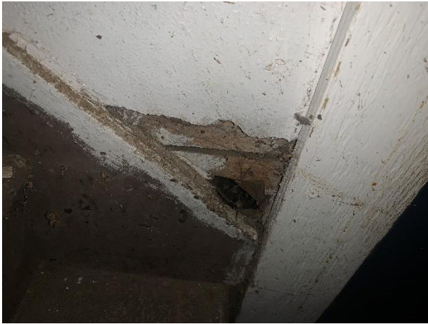
Wall Back Entry Side C
