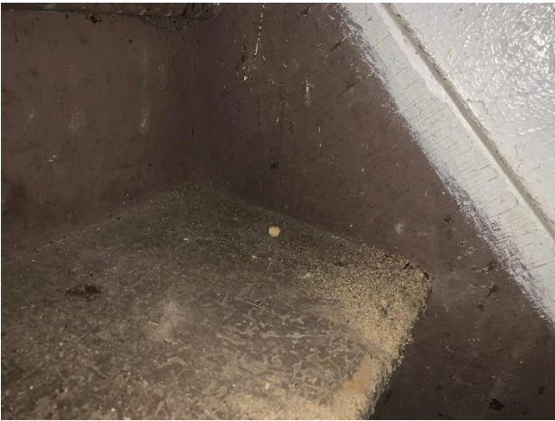
Stair Stringer Back Entry
