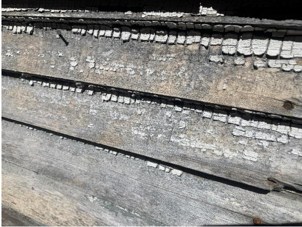
Siding Upper Porch
