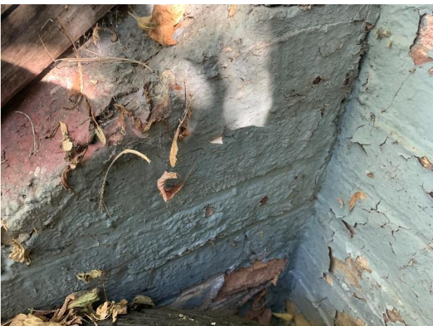
Foundation, Basement Entry Hatch Exterior Side C
