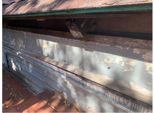
Siding Upper Porch
