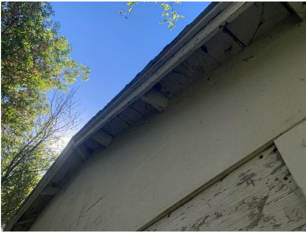
Soffit, Fascia Garage Side A
