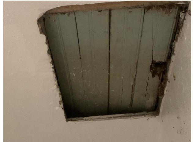
Ceiling Back Entry
