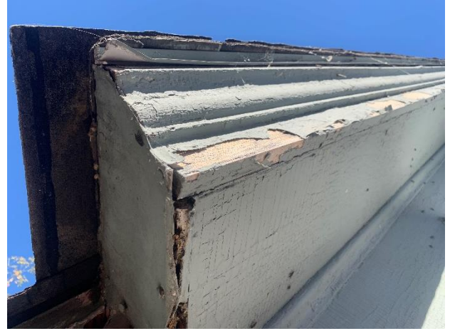
Fascia, Soffit Exterior
