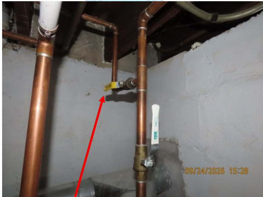
Maine water shut off for the boiler
