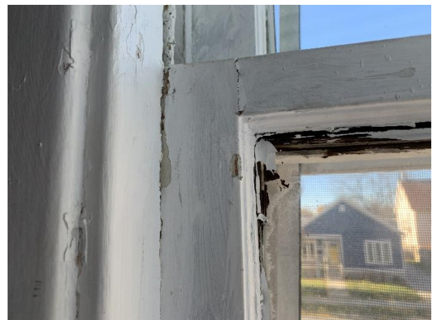
Window Sash Bedroom A
