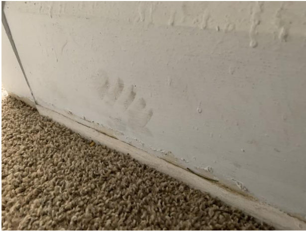
Baseboard Hallway Side D
