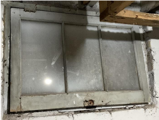
Basement Window Sash, Casing
