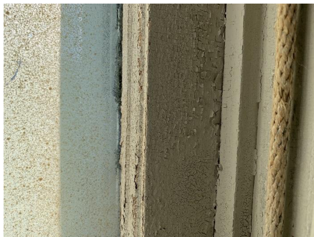
Window Sash Bedroom A Closet
