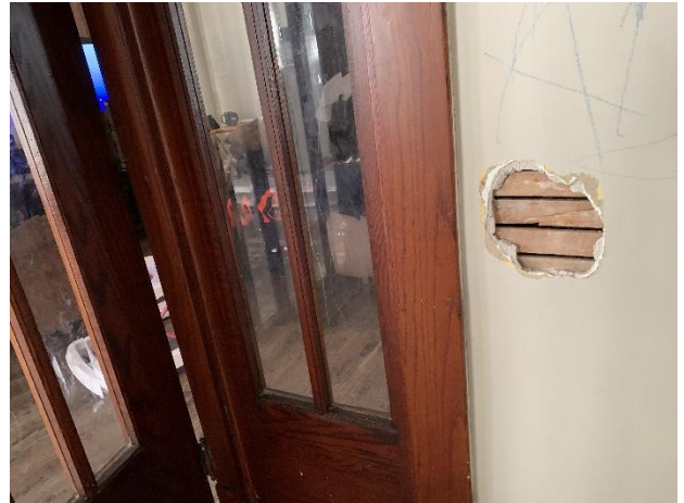
Wall Dining Room Side A
