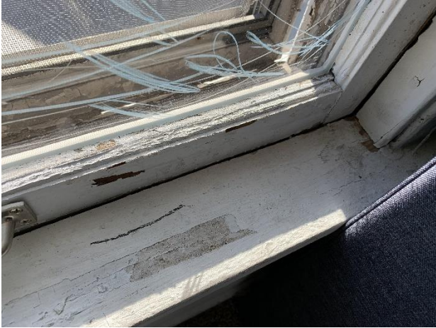
Window Sill, Sash Bedroom D
