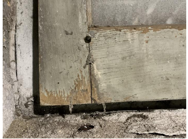
Basement Window Sash
