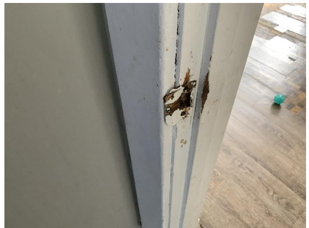
Door Jamb Lower Bathroom
