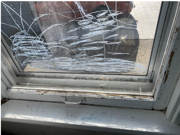
Window Sash Kitchen
