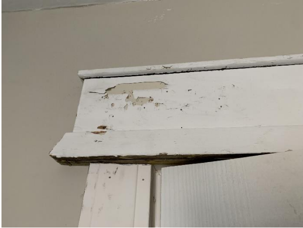
Door Casing Upper Bathroom
