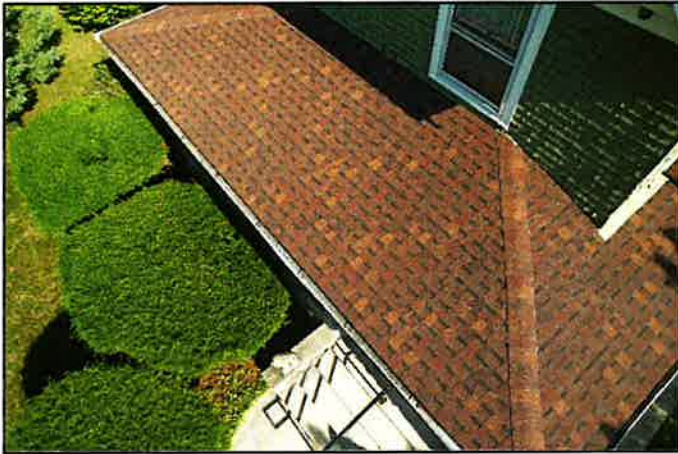
2. Asphalt shingles
