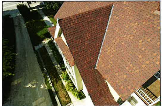
7. Asphalt shingles
