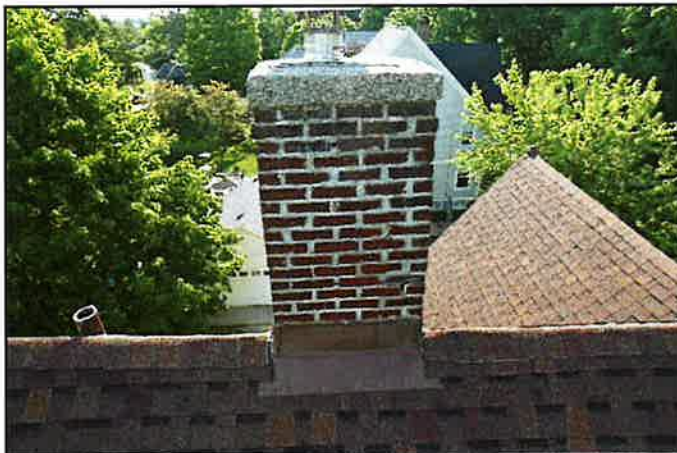
68. General photos of chimney chase
