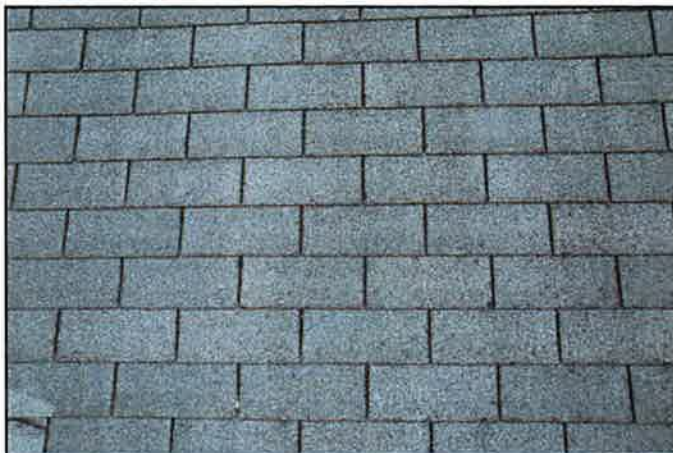
12. Asphalt shingles
