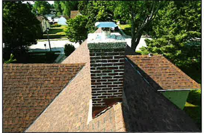
67. General photos of chimney chase
