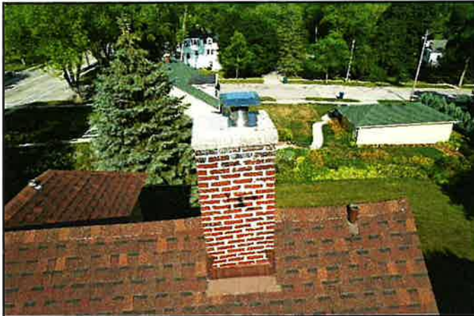
66. General photos of chimney chase
