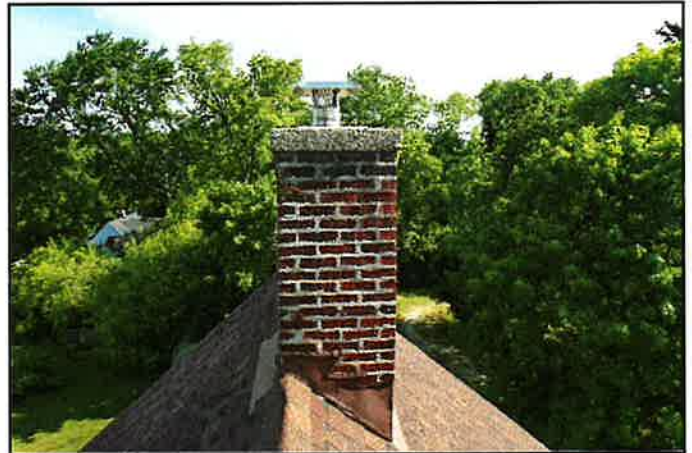
69. General photos of chimney chase
