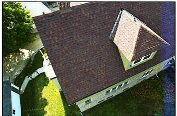
13. Asphalt shingles
