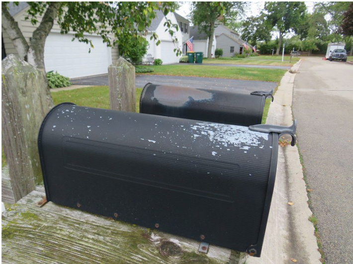
rust and finish deterioration at mailboxes
