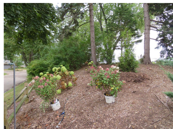
planting in process at berm
