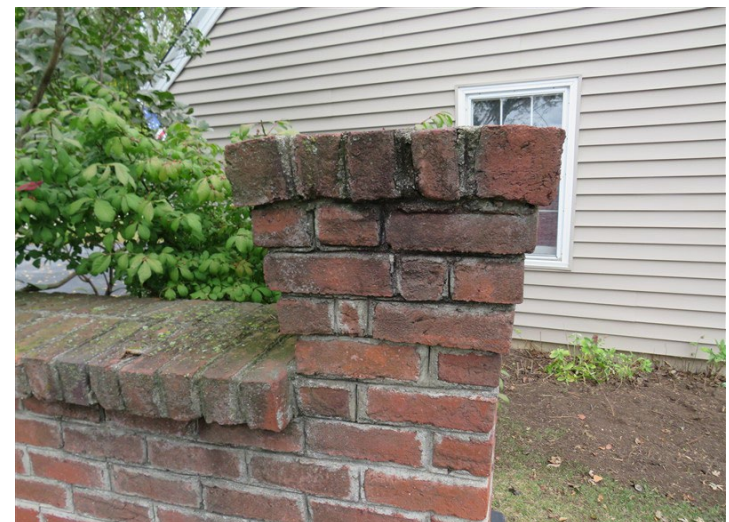
mortar deterioration
