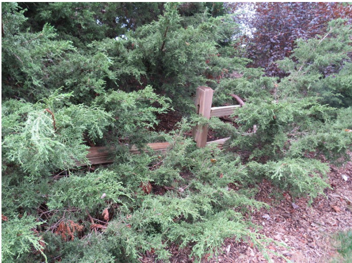
loose rail and brush overgrowing fence
