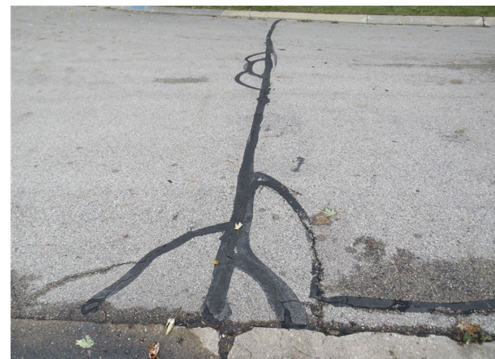
crack repairs
