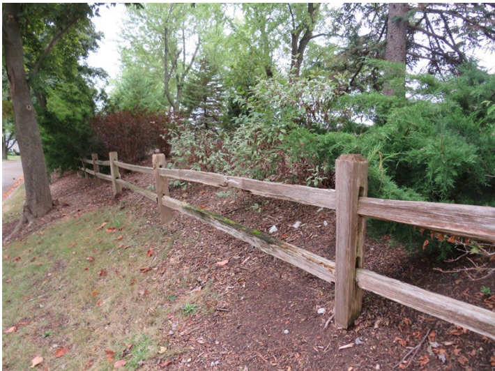
fence along berm
