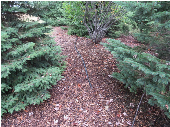
drip line at berm
