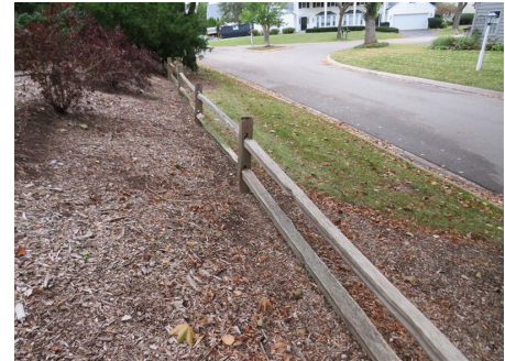
split rail fence along berm
