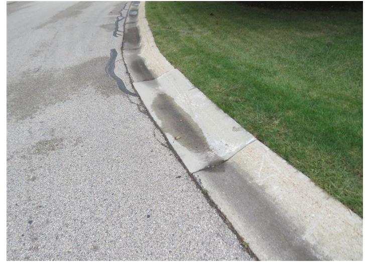
replaced section of concrete curb and gutter
