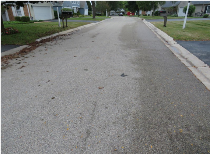
asphalt pavement at street
