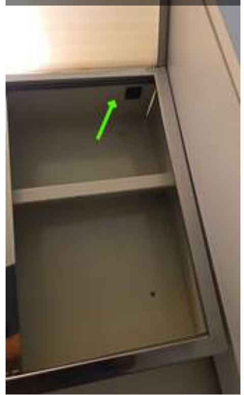
LOCATION: 1ST FLOOR HALF BATHROOM
