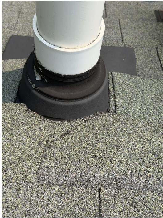
Photo 5. PVC roof penetration with rubber boot flashing.
