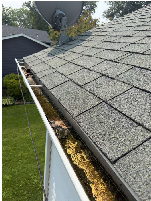
Photo 2. Standard aluminum gutter with accumulated debris and standing material.
