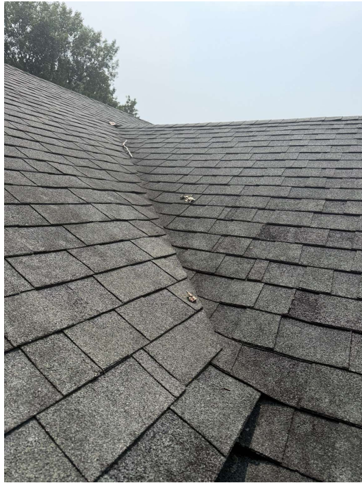
Photo 7. Roof valley and adjoining shingle surfaces.
