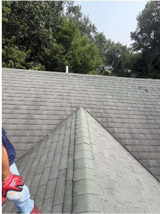
Photo 3. Overview of architectural asphalt shingles and roof planes.
