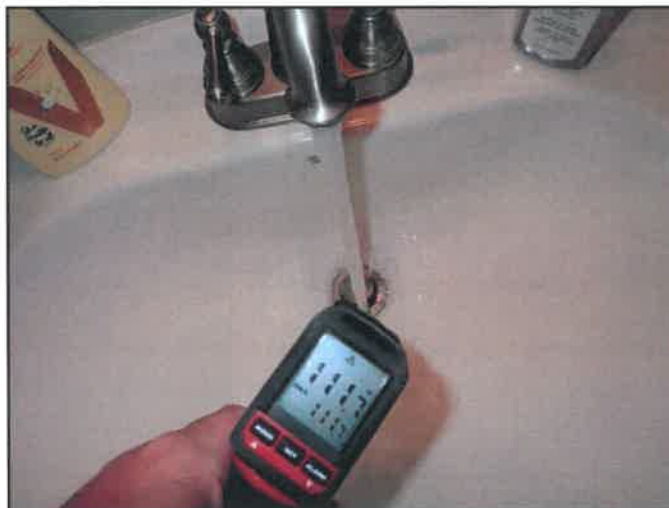
220. Service water heater
