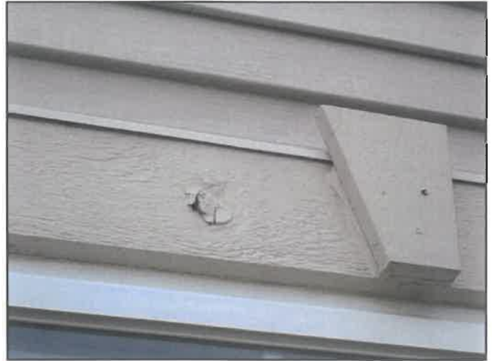
75. Rot or insect damage
