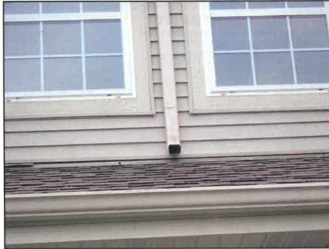
72. Discharge onto roofs
