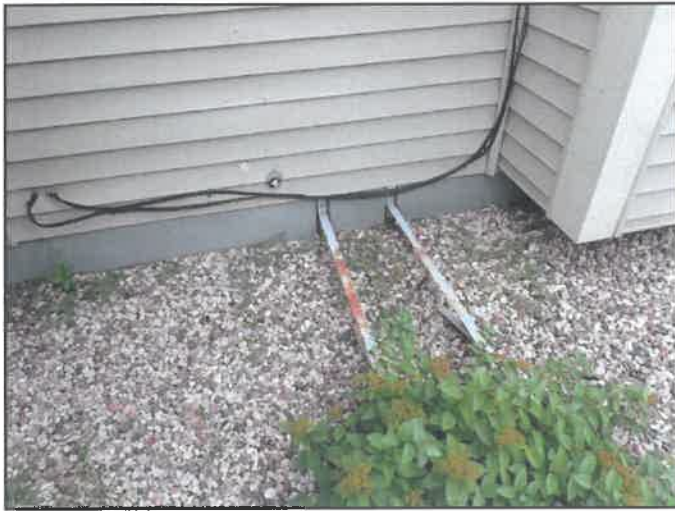
177. previous A/C location
