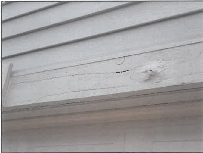
74. Rot or insect damage
