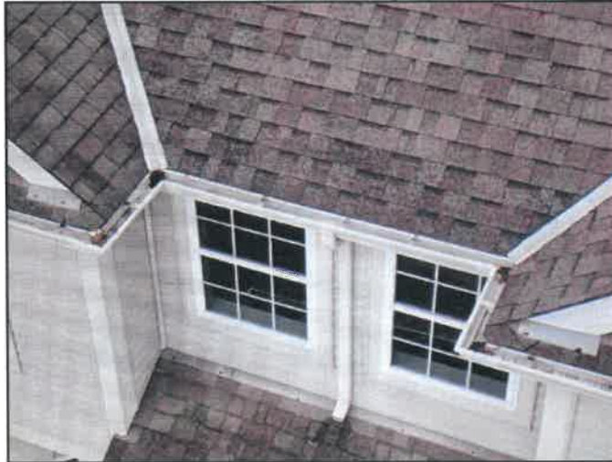
50. Inspect & repair, as needed.
