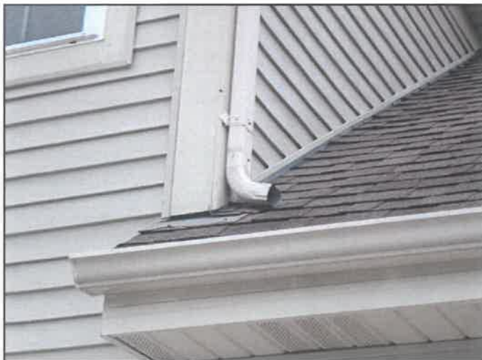
70. Discharge onto roofs
