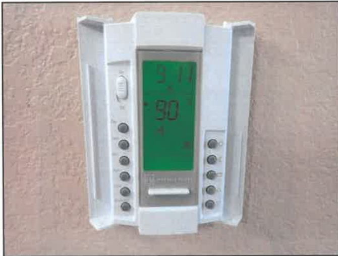
144. Radiant floor heating (electric)
