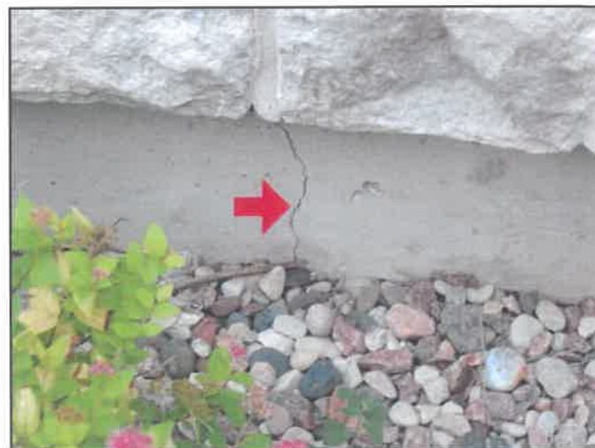
103. Cracked foundation
