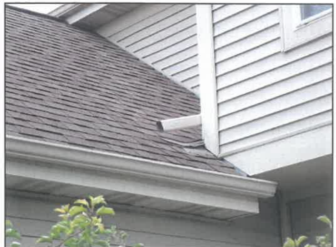
71. Discharge onto roofs
