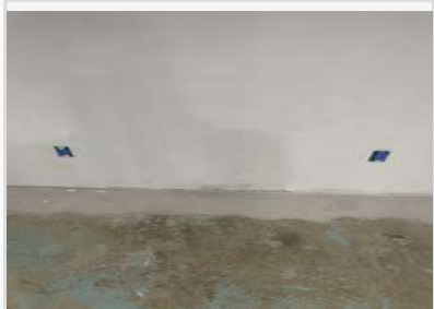
5.4.1.2 Replace cover plates after painting
