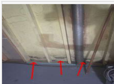
15.1.1.2 Clean mold stains at basement walls
