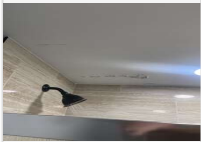
5.3.1.1 Scrape, prime, paint as needed
