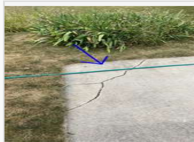
2.1.1.2 Seal cracks as needed
