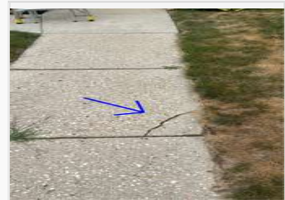
2.1.1.3 Seal cracks as needed
