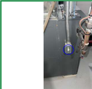
1.1 Furnace disconnect
