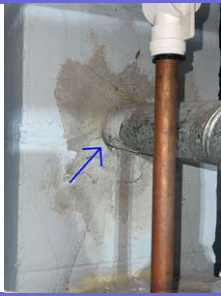
1.1 Keep areas sealed where flues enter chimney
