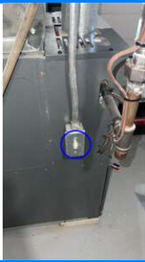
1.1 Furnace disconnect
