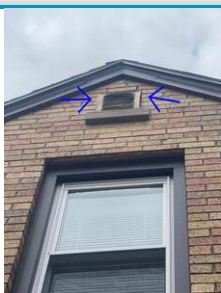
1.1 Replace caulking as needed
