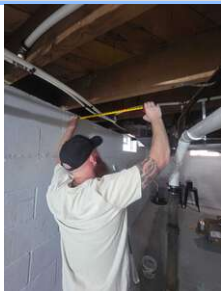
1.1 Walls showed signs of little to no movement
