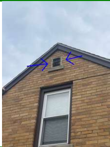
1.2 Replace caulking as needed
