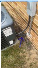
1.2 Replace foam insulation as needed
