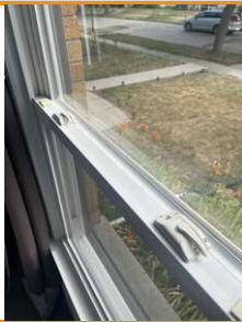
1.1 Lock hardware may need adjustment
