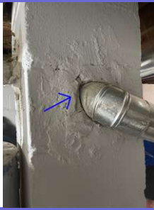
1.2 Keep areas sealed where flues enter chimney
