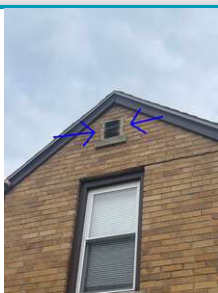
1.2 Replace caulking as needed
