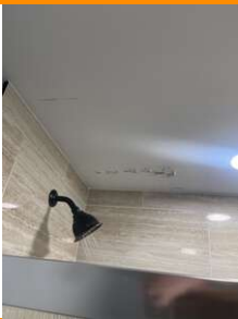
1.1 Scrape, prime, paint as needed
