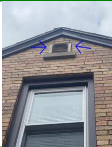
1.1 Replace caulking as needed
