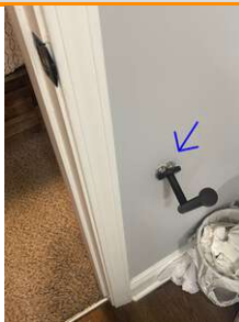
1.3 Repair as needed
