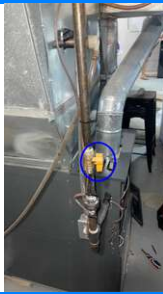
1.2 Furnace gas shut off
