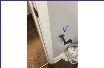
1.3 Repair as needed
