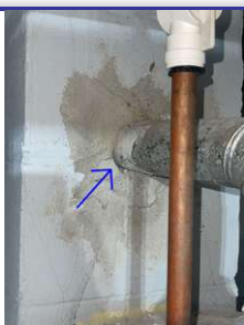
1.1 Keep areas sealed where flues enter chimney
