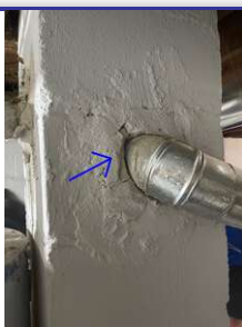
1.2 Keep areas sealed where flues enter chimney
