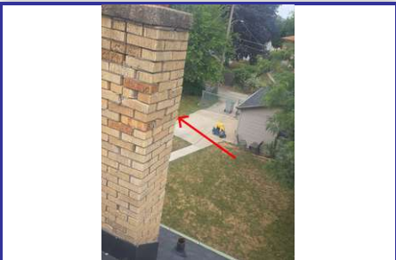
1.2 Repair any damaged/open joints at chimney
