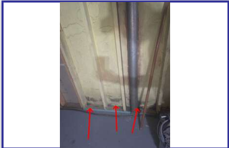
1.1 Clean mold stains at basement walls
