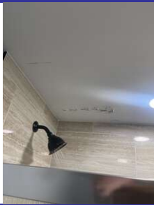
1.1 Scrape, prime, paint as needed
