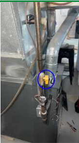
1.2 Furnace gas shut off
