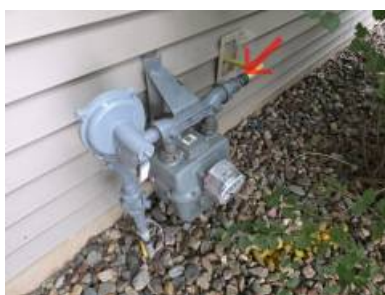
GAS SERVICE LINE AND OUTDOOR METER
