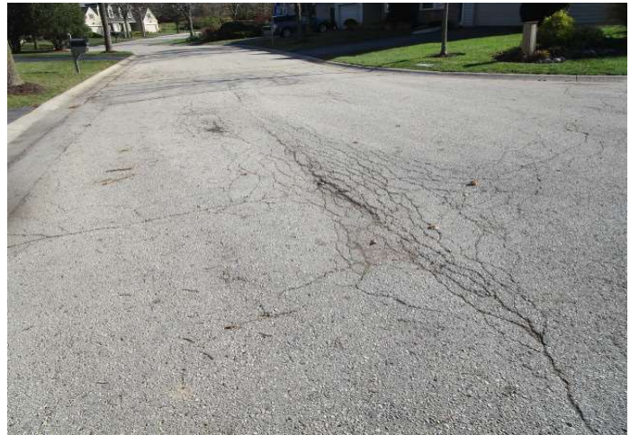
Fatigue cracks
