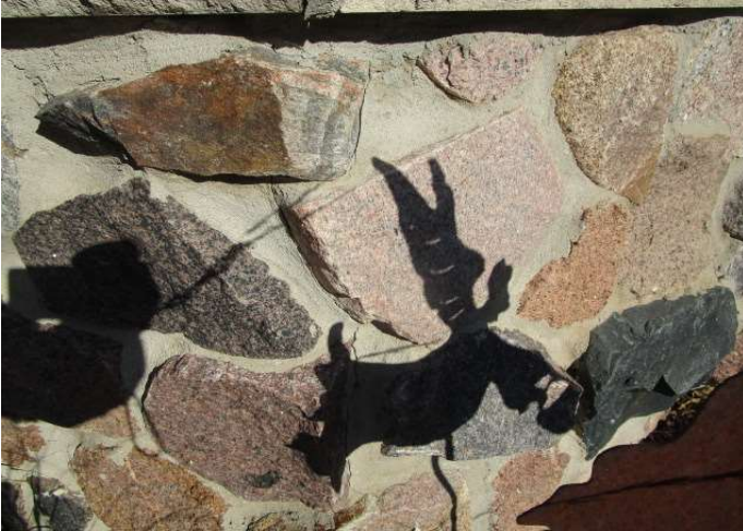
Mortar crack
