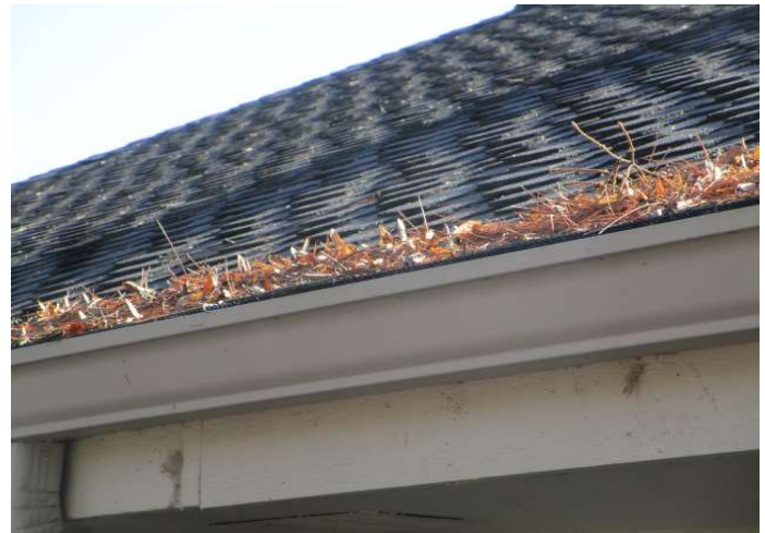
Leaf guard filled with debris
