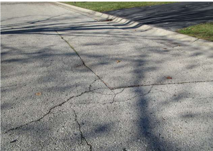
Fatigue cracks
