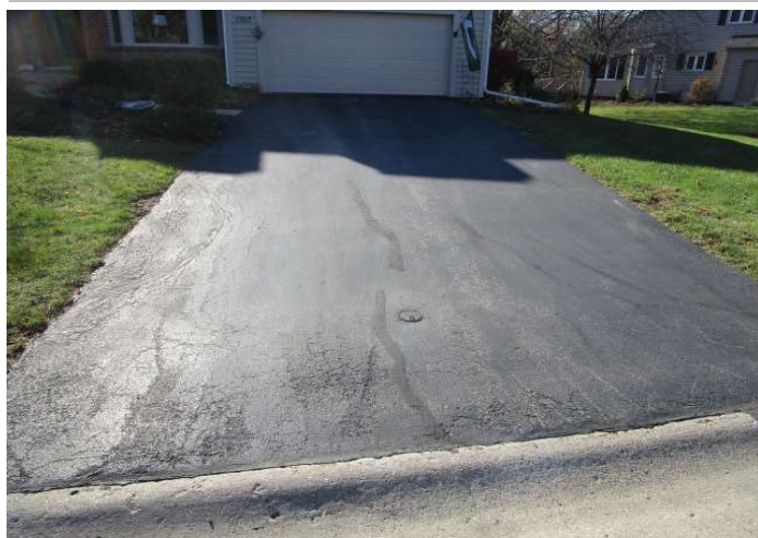
Driveway overview with areas of crack fill
