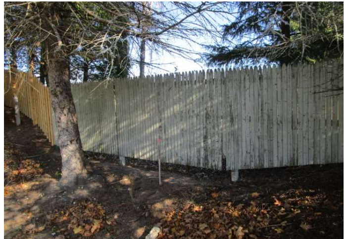
Older sections of fencing
