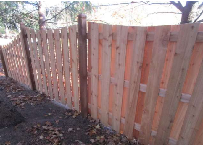
East perimeter fence overview
