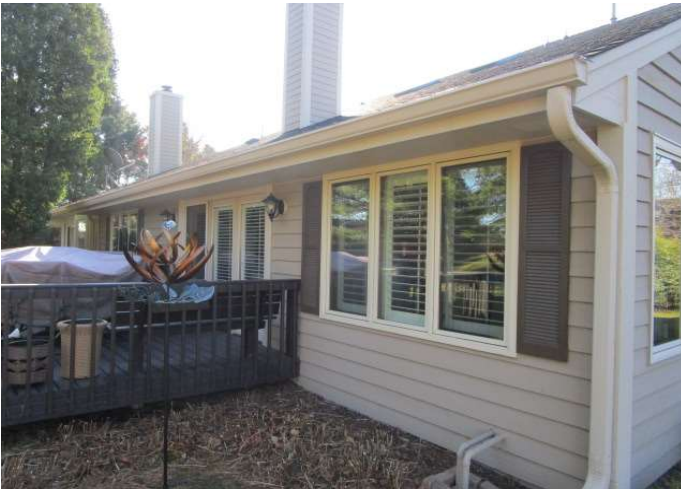
Gutter and downspout overview
