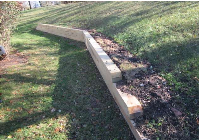
Short timber retaining wall 2 of 2
