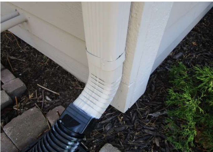
Downspout detail view
