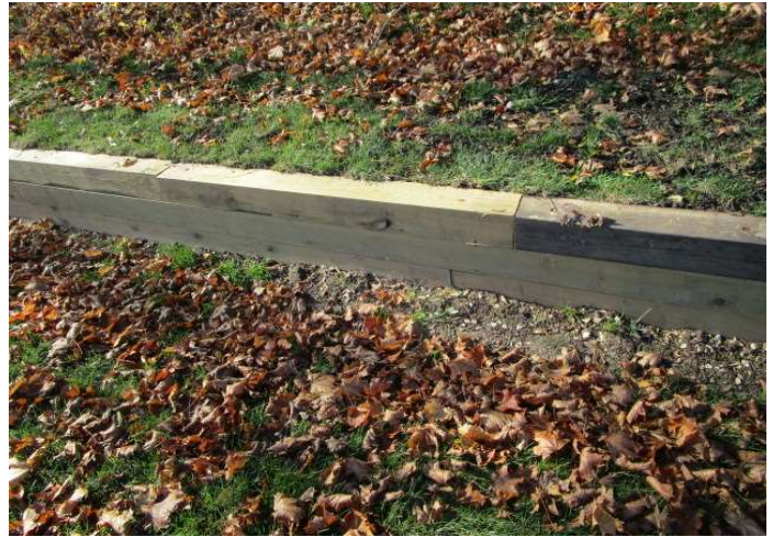
Short timber retaining wall 1 of 2
