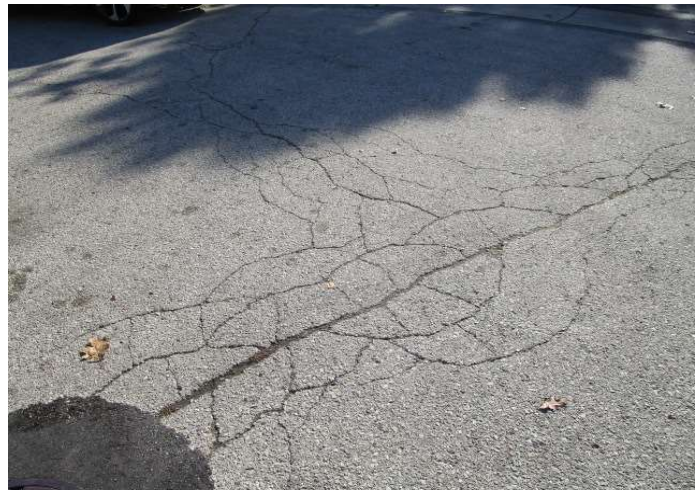
Fatigue cracks
