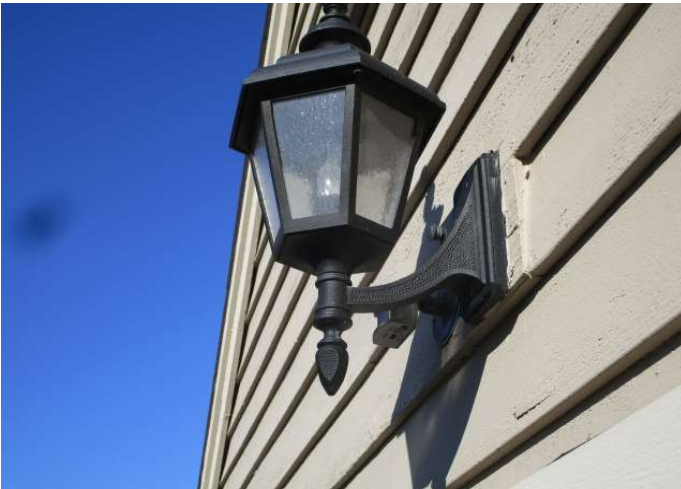
Single large sconce over a garage door
