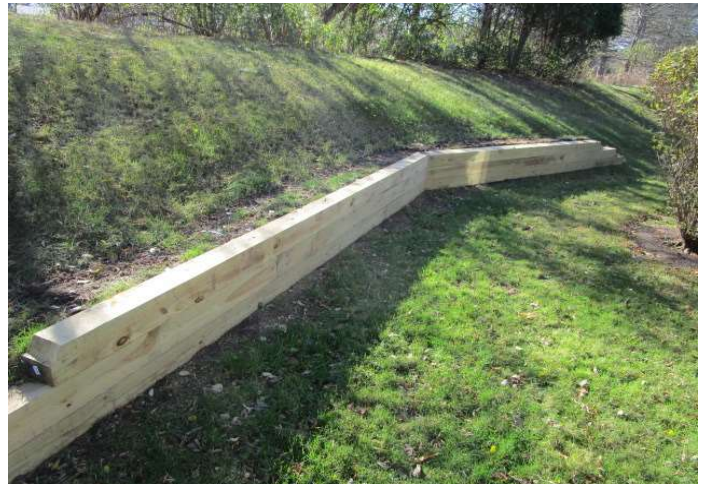
Short timber retaining wall 2 of 2
