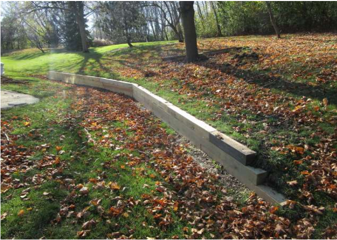
Short timber retaining wall 1 of 2
