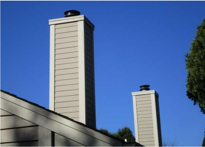
Chimney caps overview
