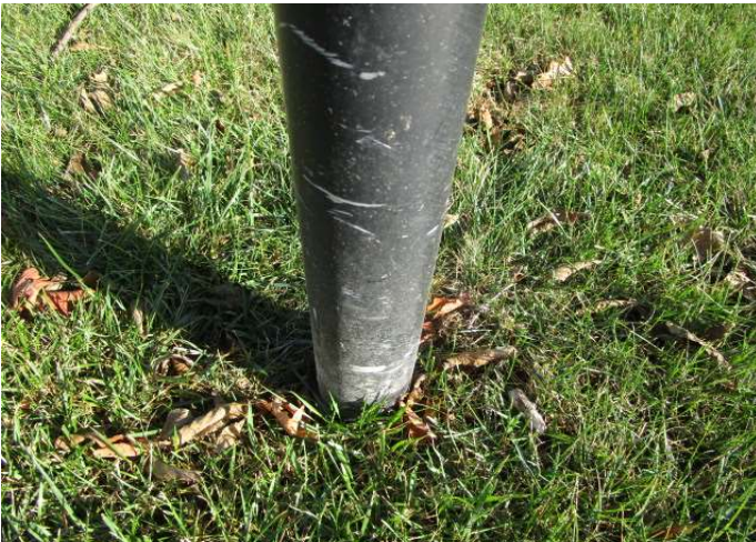
Light pole detail view
