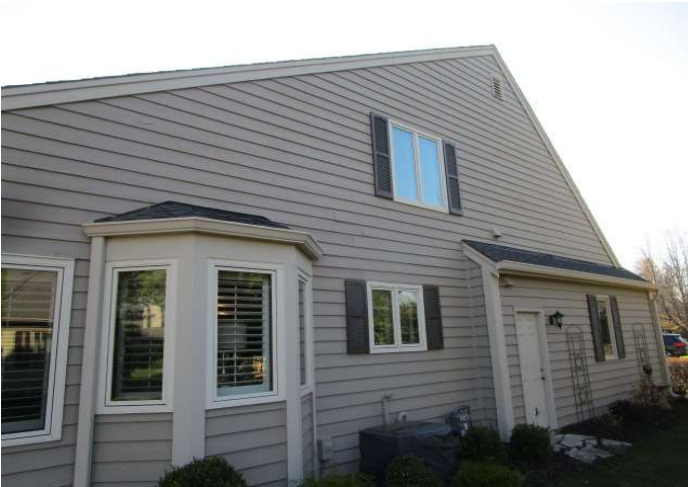
Painted exterior surfaces overview
