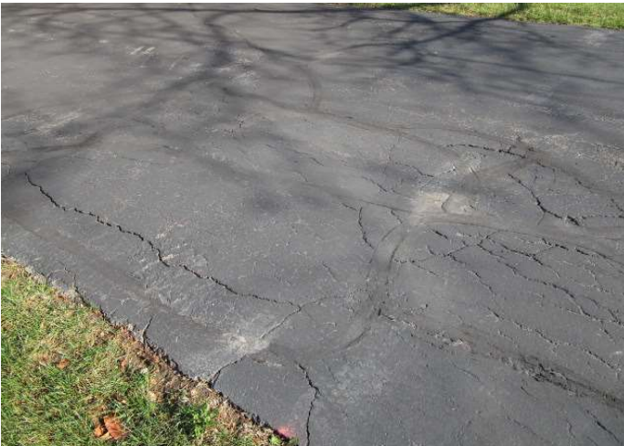
Fatigue cracks
