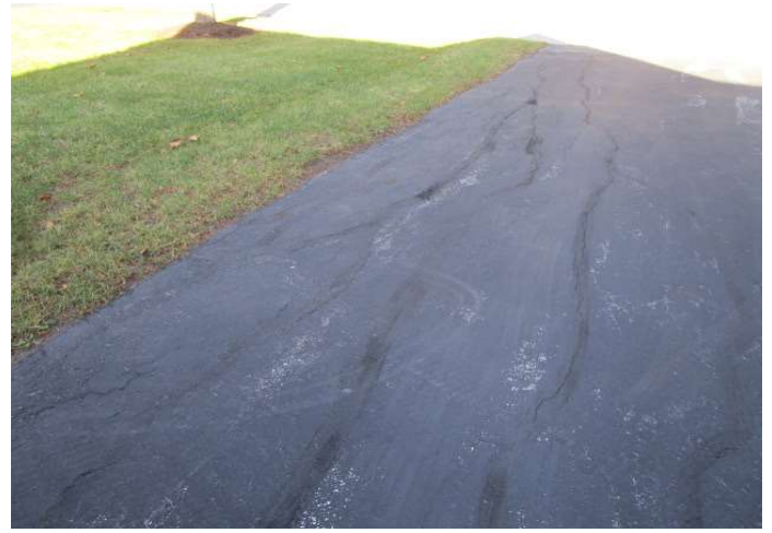
Various crack fill
