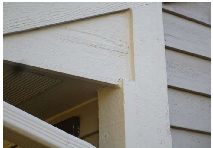
Wood soffit and fascia
