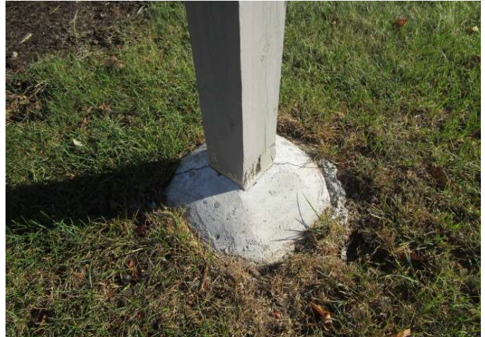
Post is set in concrete
