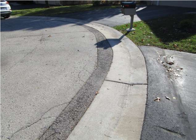
Newer curb at Pinewood Court
