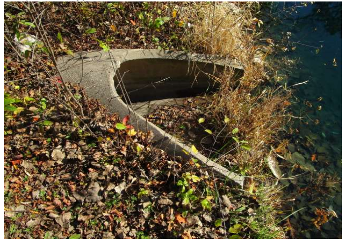
Inlet structure at the south pond
