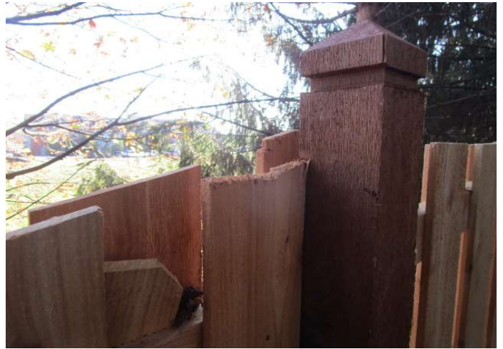
Fence detail view
