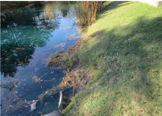
Eroded shoreline at the north pond
