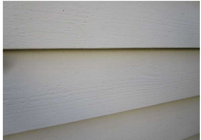
Cedar lap siding detail view in good condition
