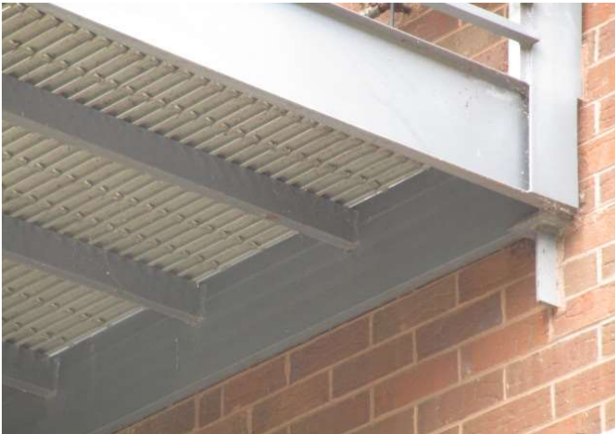
Floor grating at unit balcony
