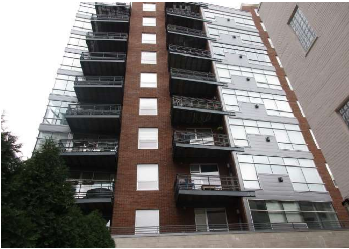
Overview of metal balcony structures
