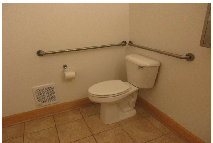
Toilet and grab bars
