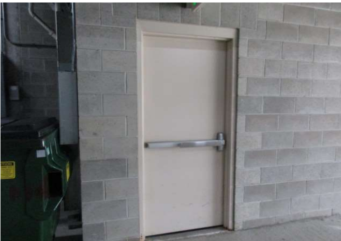
Metal door at parking garage
