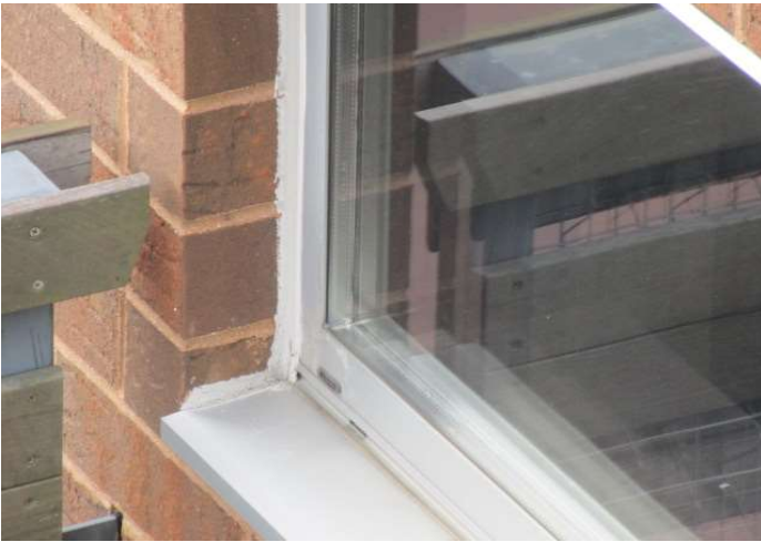
Sealant at window perimeter, viewed from roof
