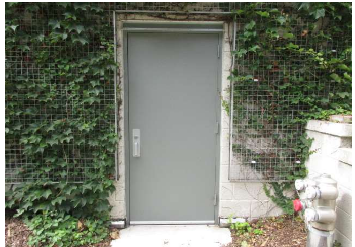
Exterior door at community room - recently replaced
