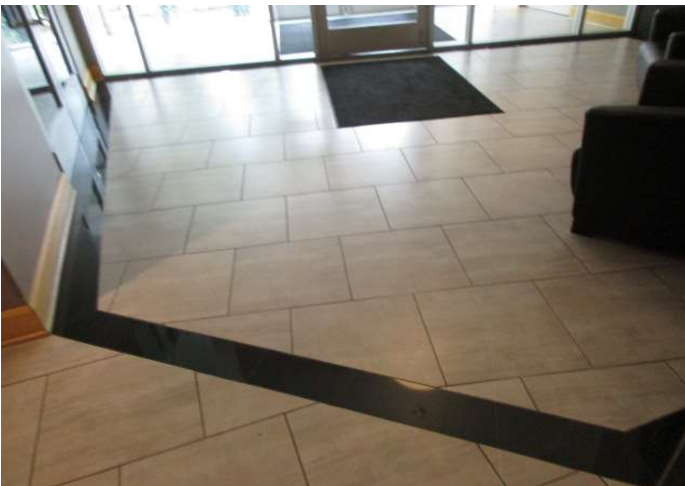
Tile flooring at lobby
