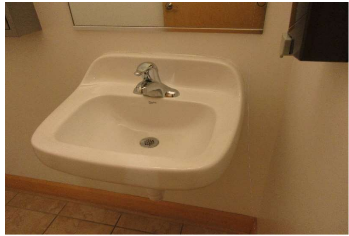
Wall-hung ADA compliant sink
