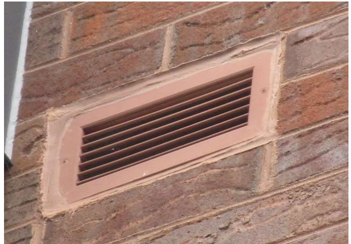
Sealant at perimeter of wall vent
