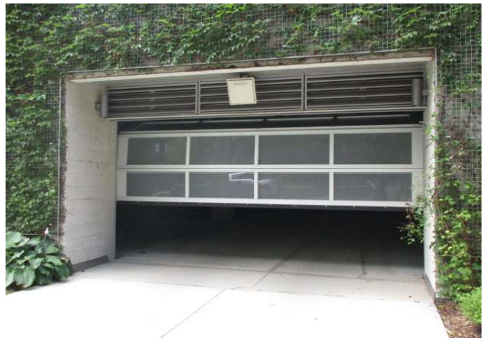
Garage door, replaced 2018
