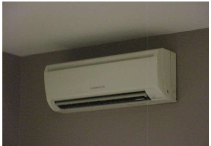
Typical indoor wall-mounted evaporator / blower unit
