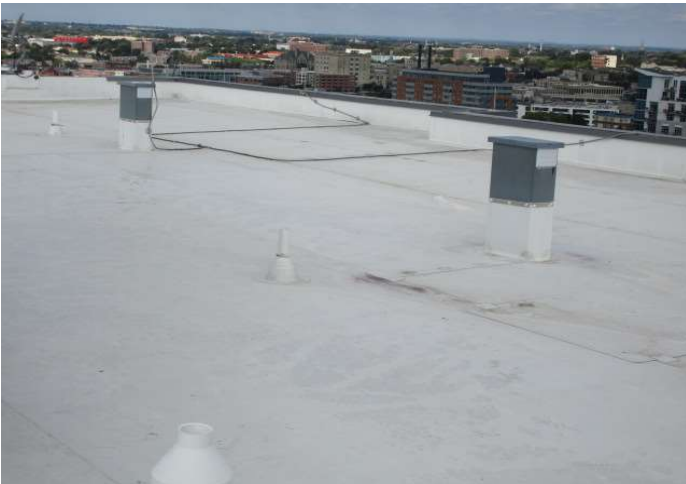
Overview of roof membrane
