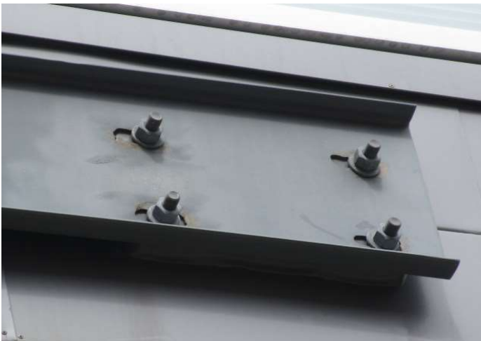
Paint finishes at metal balcony structure
