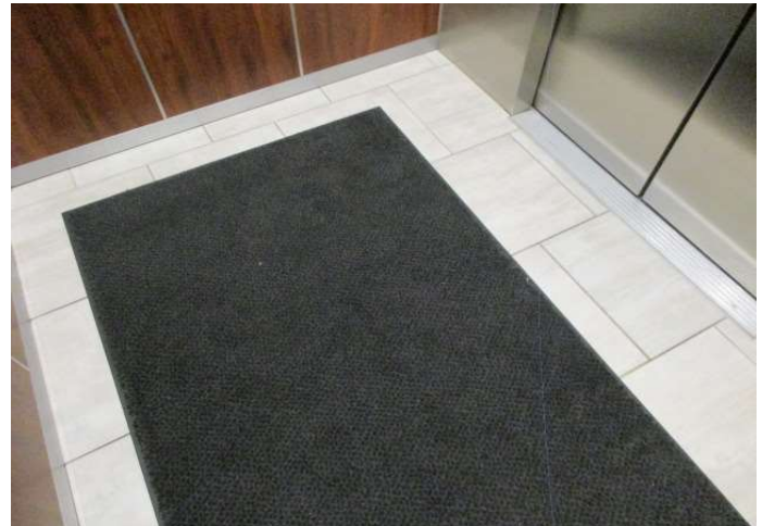
Tile floor at elevator cab
