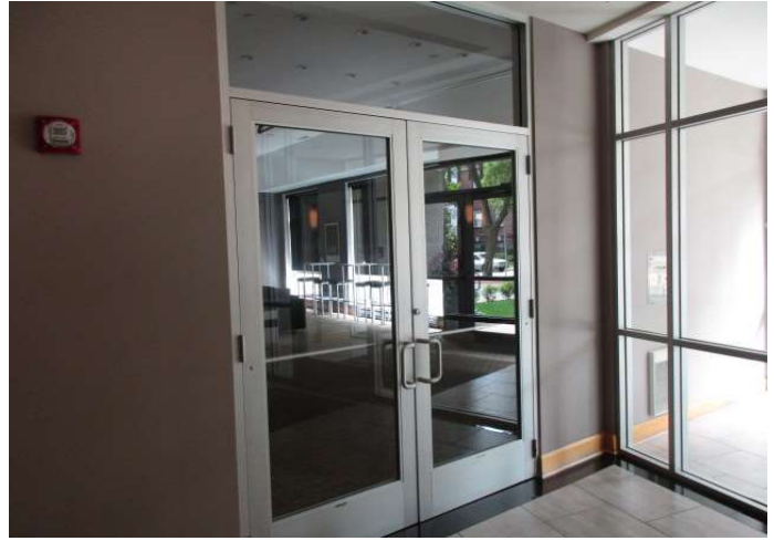
Community room doors and vestibule glazing
