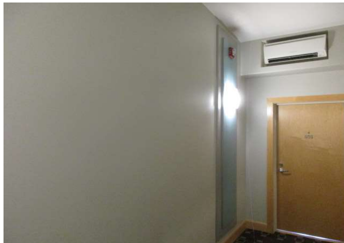
Paint finishes at interior walls and ceiling
