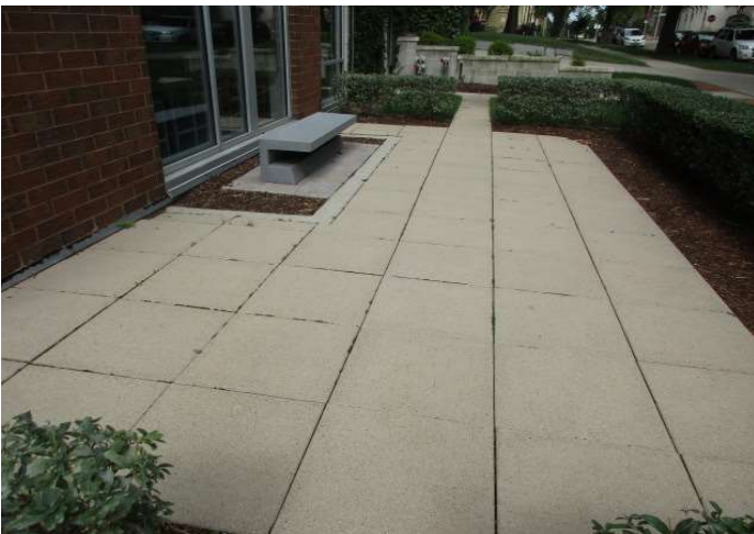
Concrete pavers at Community Room patio
