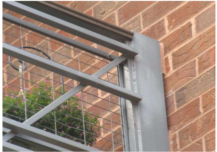
Typical railing at unit balcony
