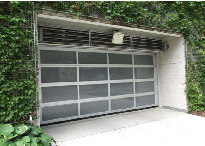
Garage door, replaced 2018
