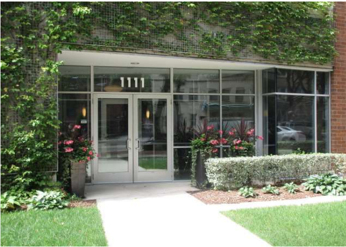
Windows and glass doors at main entrance
