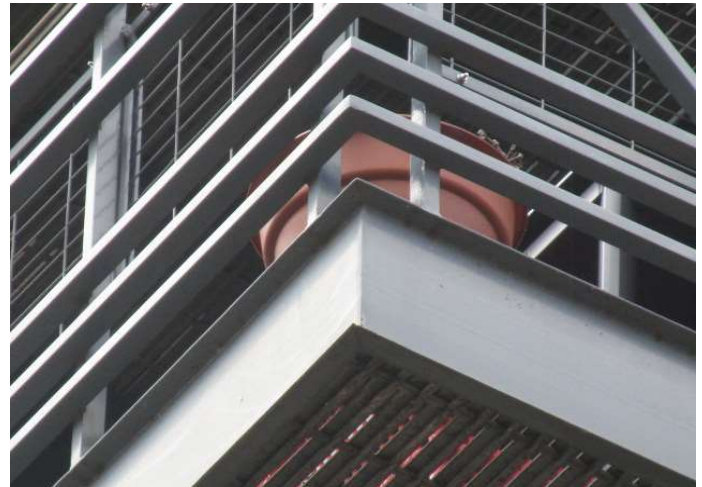
Paint finishes at metal balcony structure
