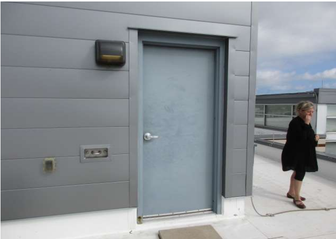
Exterior metal door at roof level
