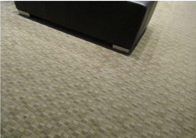
Carpet flooring at Community Room
