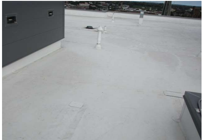
Overview of roof membrane
