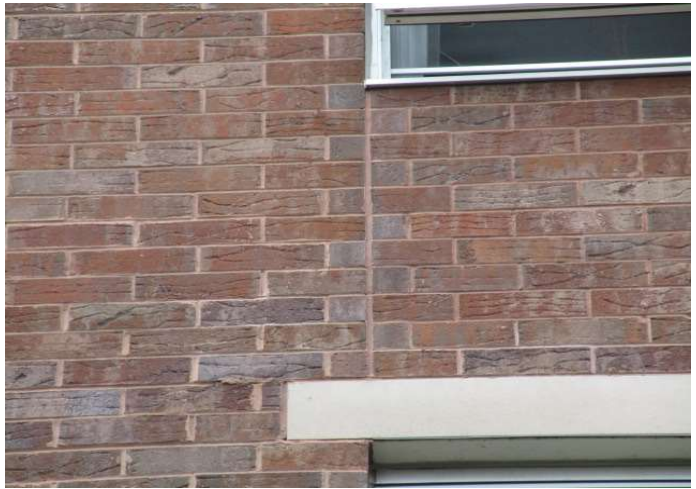
Brick masonry façade, with control joint
