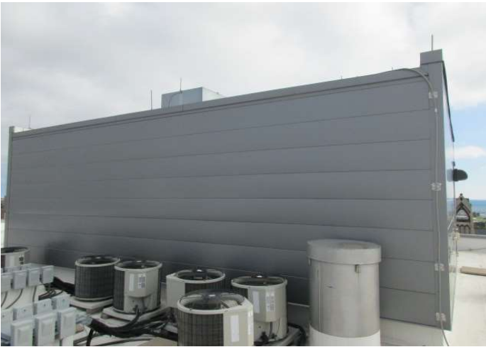
Aluminum siding at rooftop stairwell penthouse
