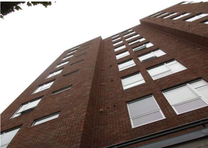
Overview of masonry façade
