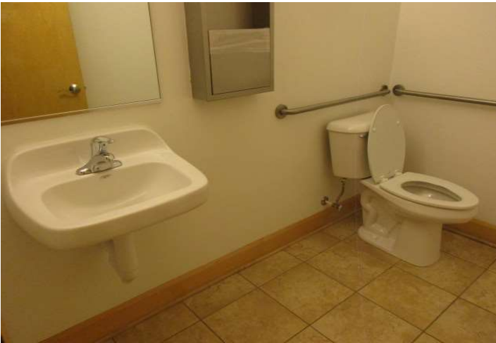
Overview of common rest room at 1st floor
