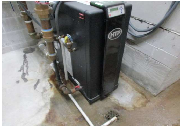
Boiler for domestic hot water
