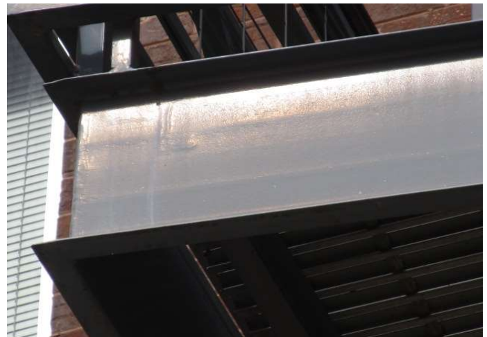
Paint finishes at metal balcony structure
