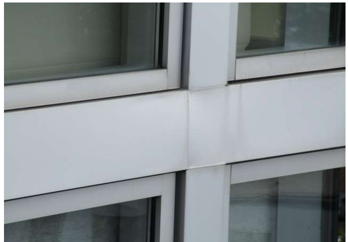
Aluminum trim at floor-to-floor
