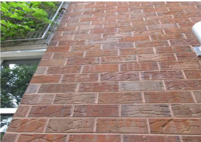
Typical condition of brick masonry façade
