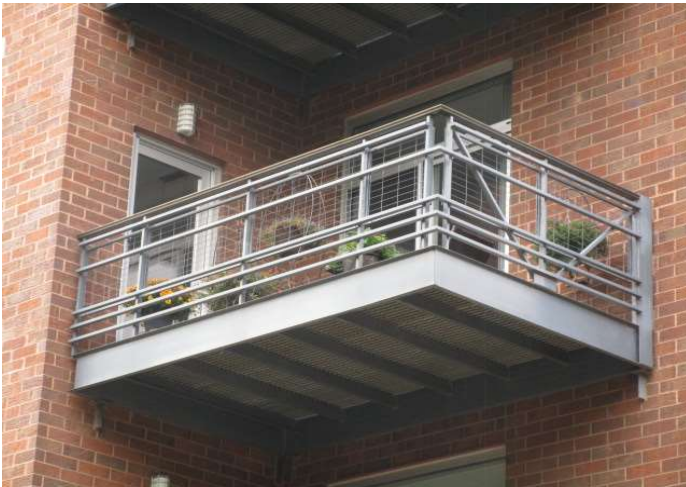
Overview of metal balcony structure
