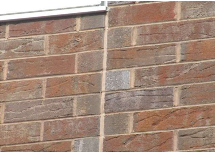
Sealant at masonry control joint
