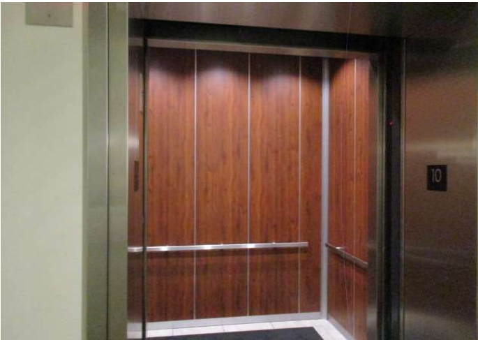
Elevator cab interior
