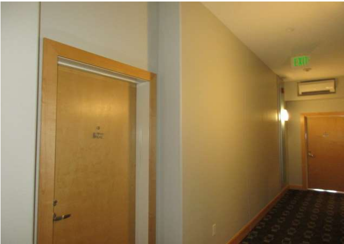
Paint finishes at interior walls and ceiling
