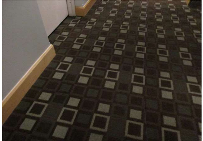
Carpet flooring at hallway
