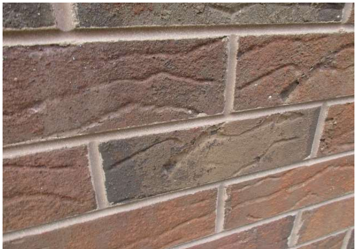
Typical condition of brick masonry façade
