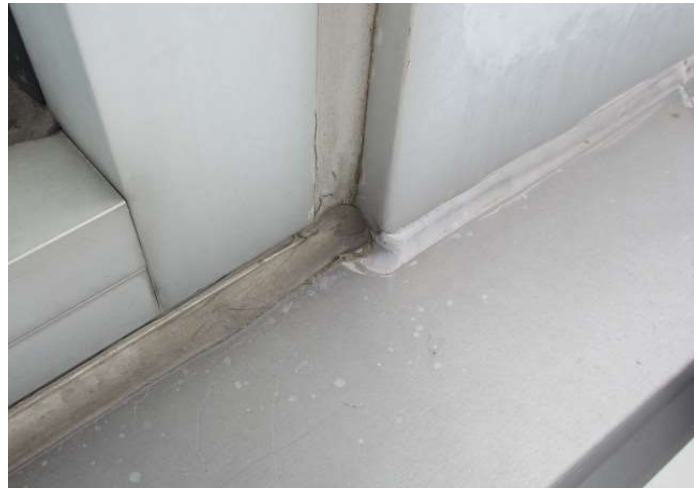
Sealants at metal-to-metal joints
