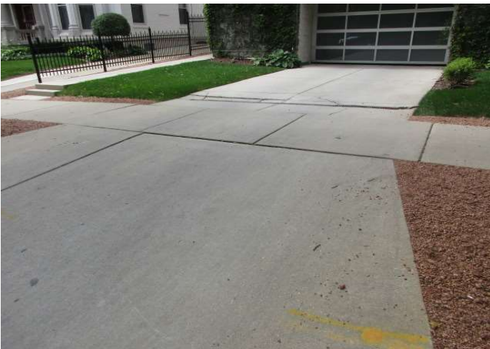
Concrete driveway and apron
