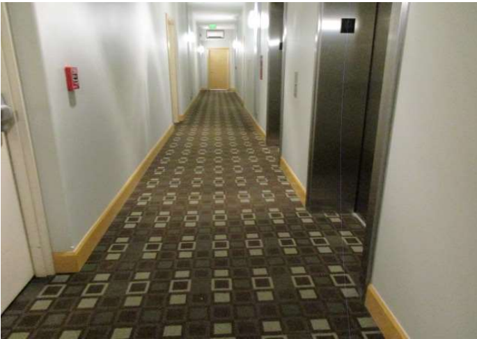
Carpet flooring at hallway
