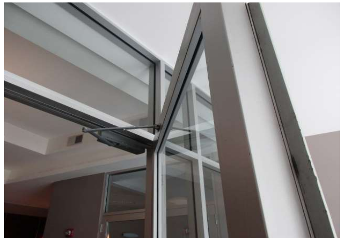
Door frame at interior of vestibule
