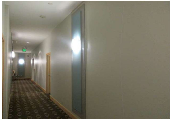
Laminate wall features at hallway
