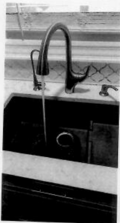
Countertops and Cabinets: Inspected Cabinets and Countertops
