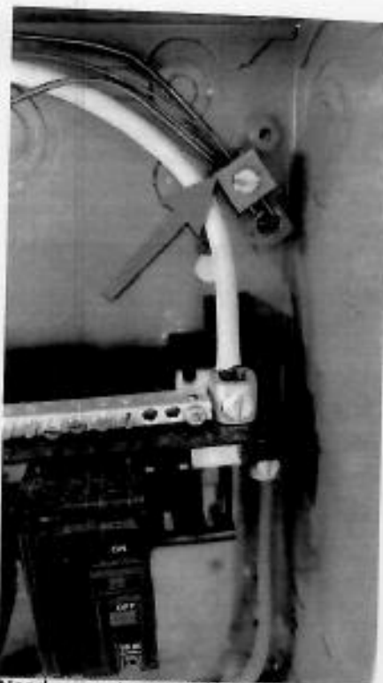
Need separate ground bar and separated
