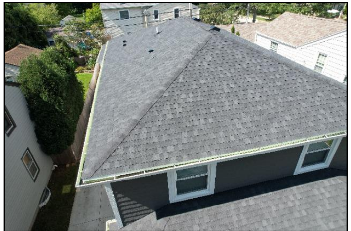
2. Asphalt shingles
