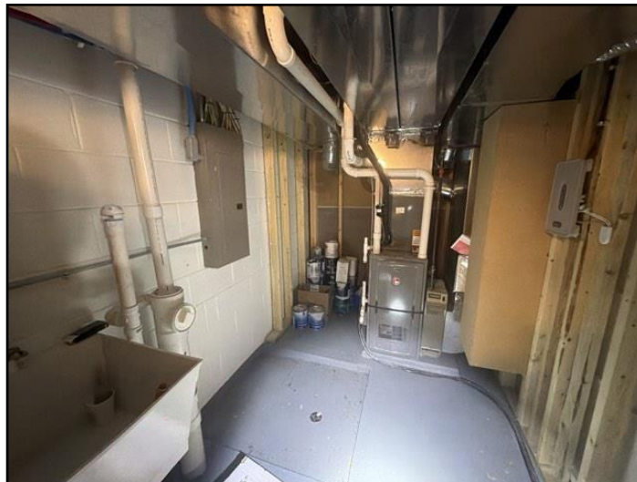
31. Ceiling, wall and floor coverings
