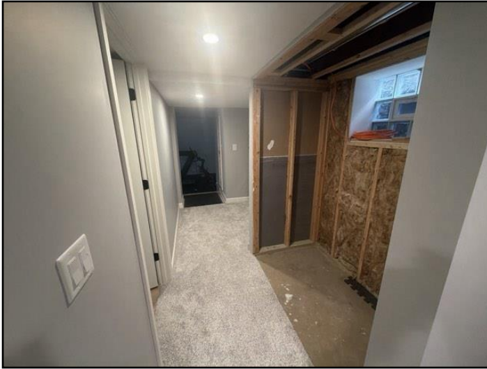
25. Ceiling, wall and floor coverings
