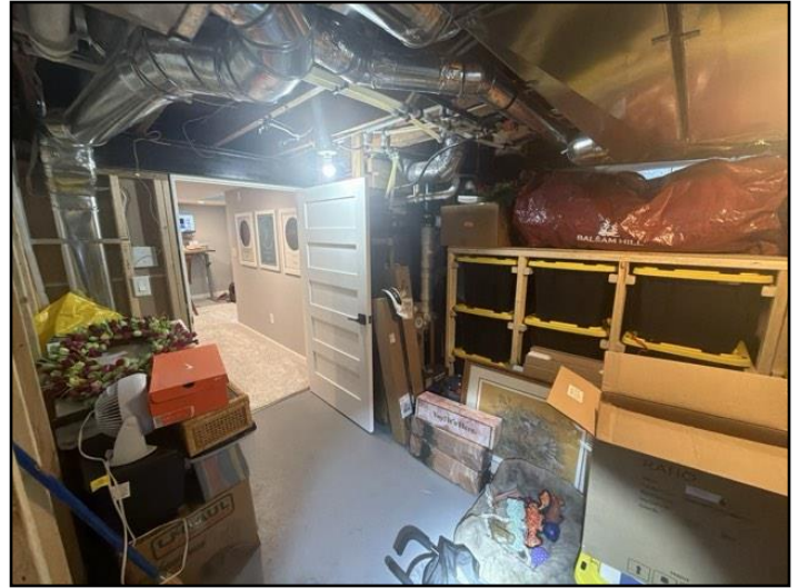
30. Ceiling, wall and floor coverings
