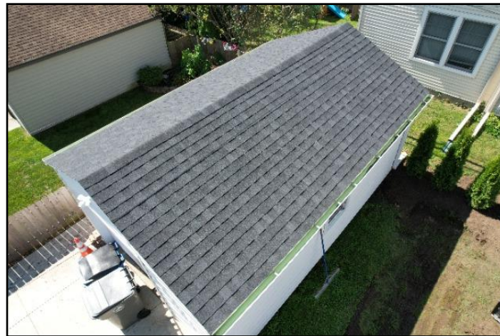
13. Asphalt shingles
