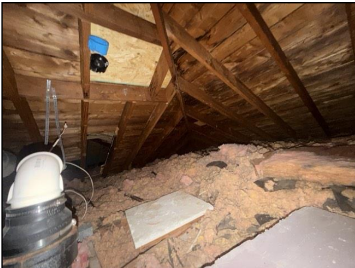
34. Inspected from access hatch
