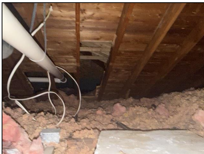
36. Inspected from access hatch
