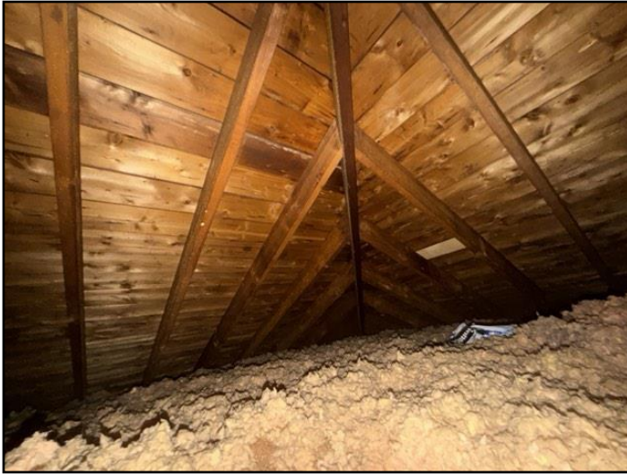
32. Inspected from access hatch
