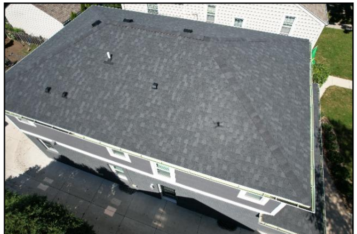
10. Asphalt shingles
