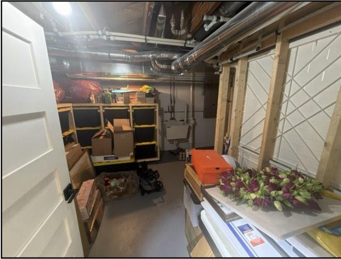
29. Ceiling, wall and floor coverings
