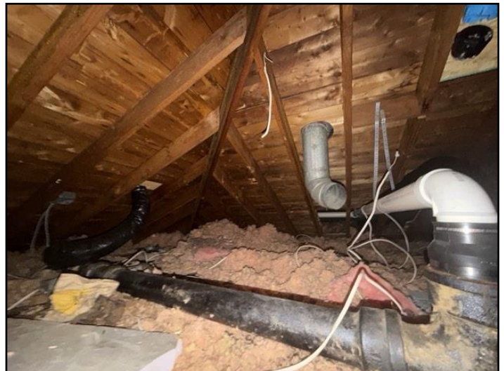
35. Inspected from access hatch
