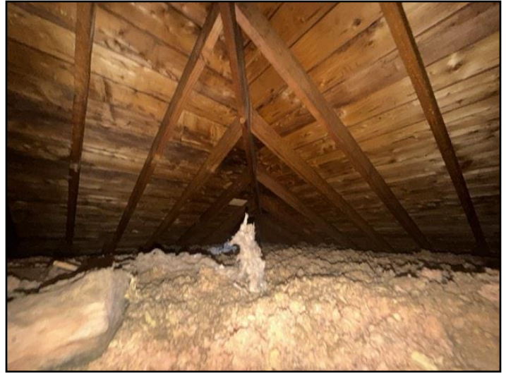
33. Inspected from access hatch
