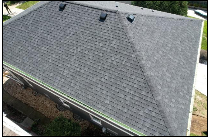
6. Asphalt shingles
