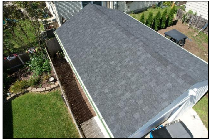
12. Asphalt shingles
