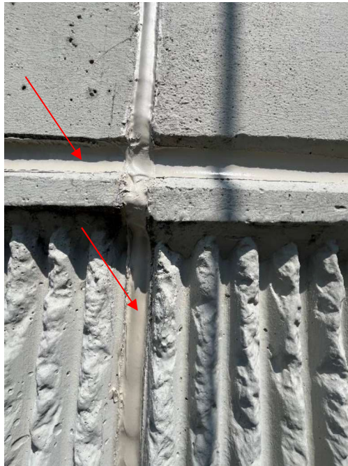
1- De-bonded sealant joint repairs- Sealant was removed and replaced with a new sealant
