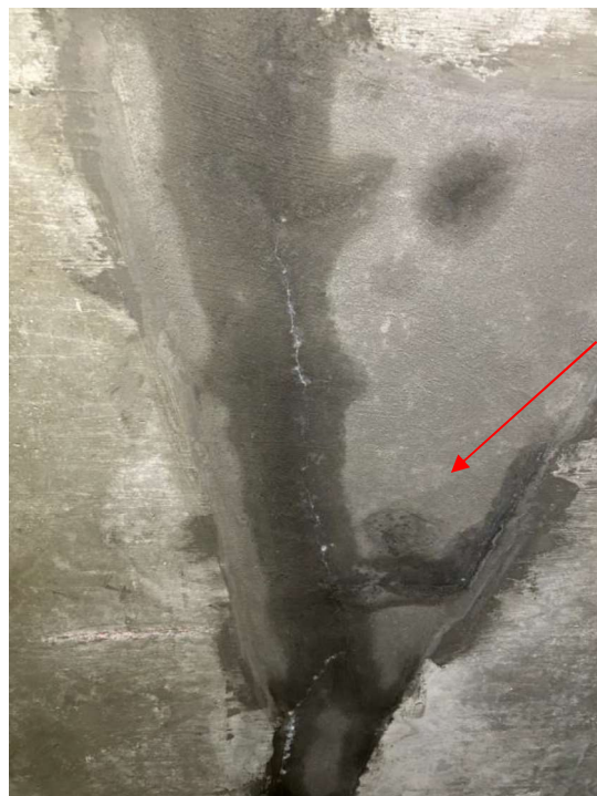
5B- Spalled concrete, more than 1-1/2 inches deep repairs - the spalled concrete area was investigated, existing steel was protected, concrete was squared, and a concrete patch was installed.
