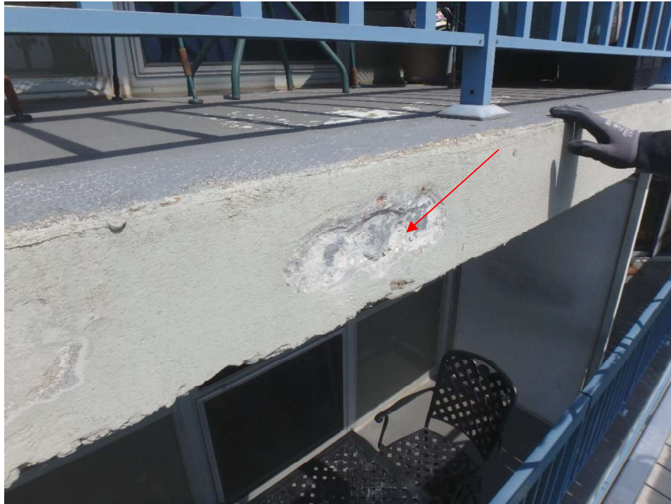
6- Concrete pocket repairs at post-tensioned concrete deck balconies- Unsound concrete was removed, PT-end protected and pocked sealed and painted
