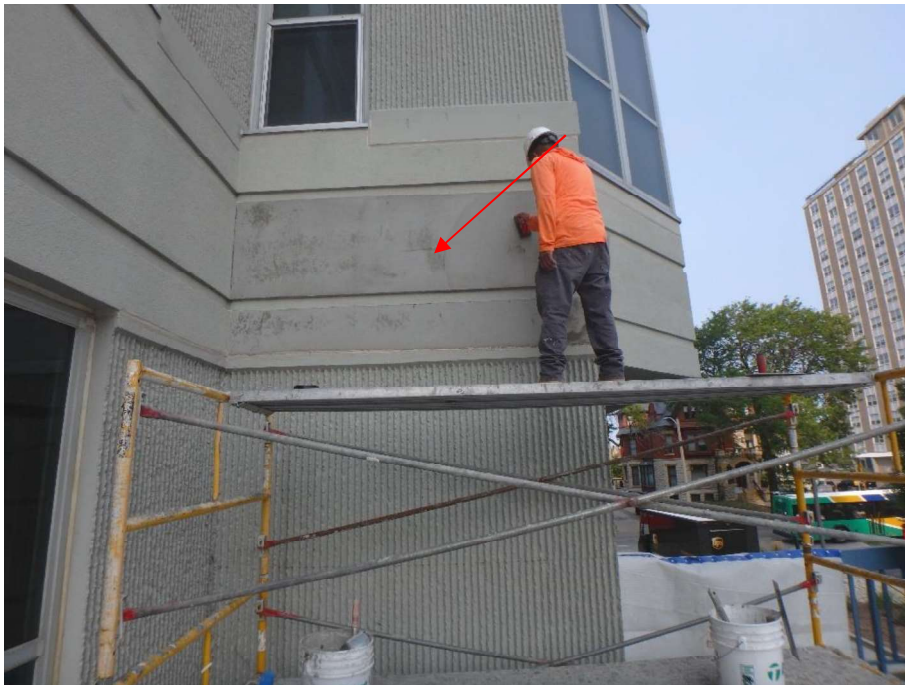
4- EIFS Repairs- Materials in the damaged areas were removed and replaced
