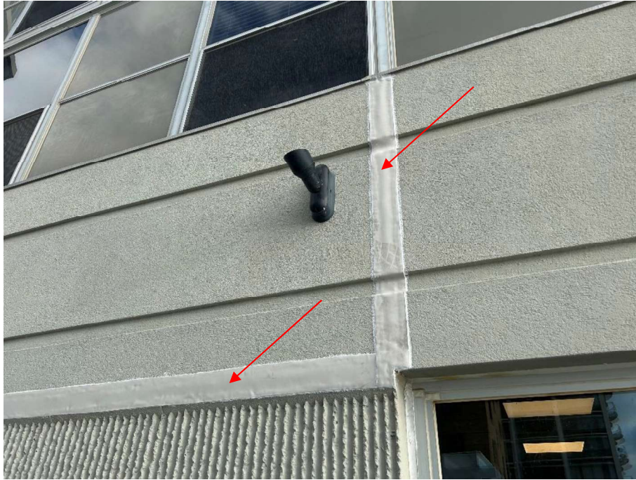
3- EIFS deteriorated sealant repairs - Deteriorated sealant was removed and replaced with new backer rod and sealant or silicon extrusions installed.
