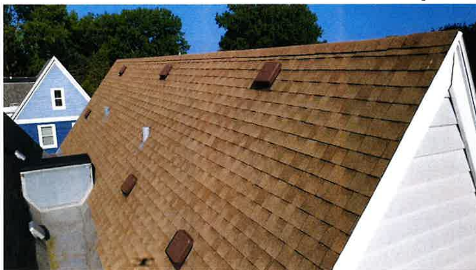
Roof photo for your reference
