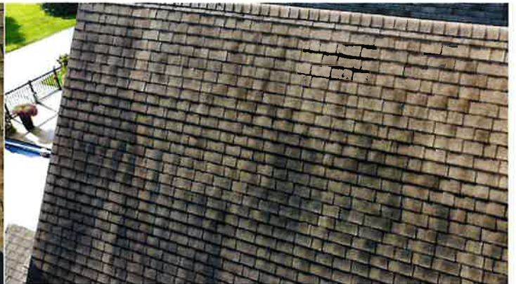
Roof photo for your reference
