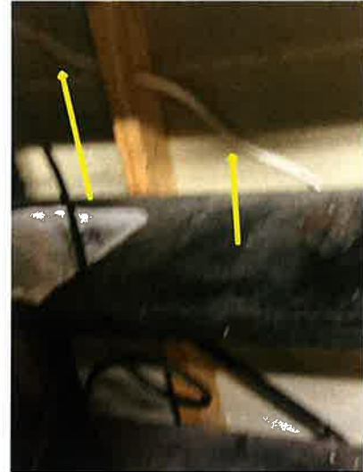
Cover horizontal wiring and stud cavities
