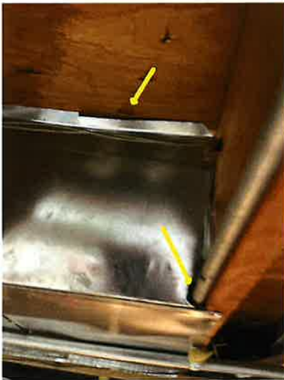
Seal return air ducts where needed.
