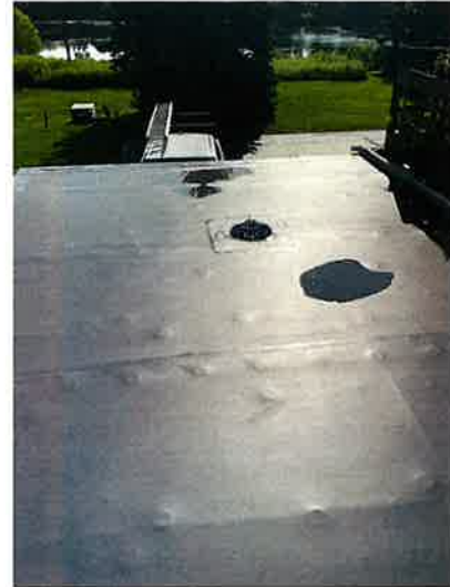
New flat roof
