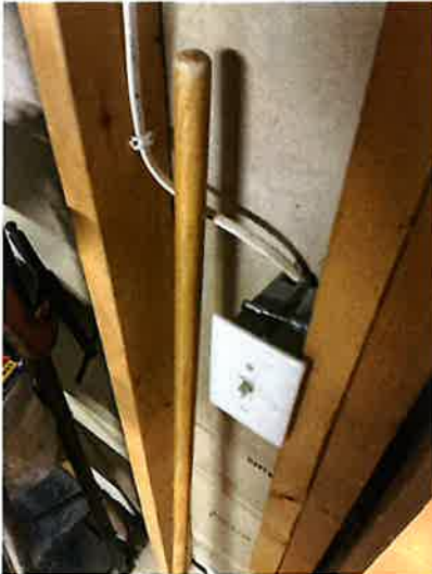
Cover horizontal wiring and stud cavities
