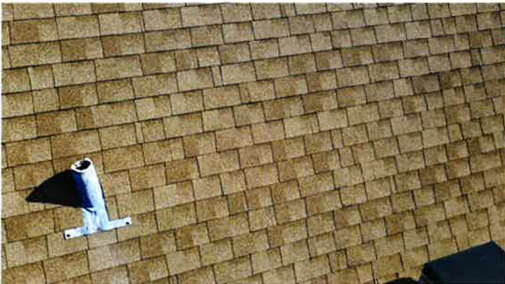
Roof photo for your reference
