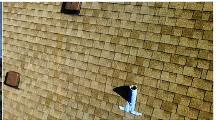
Lead flashing satisfactory
