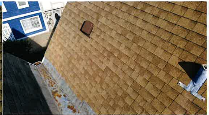
Roof photo for your reference
