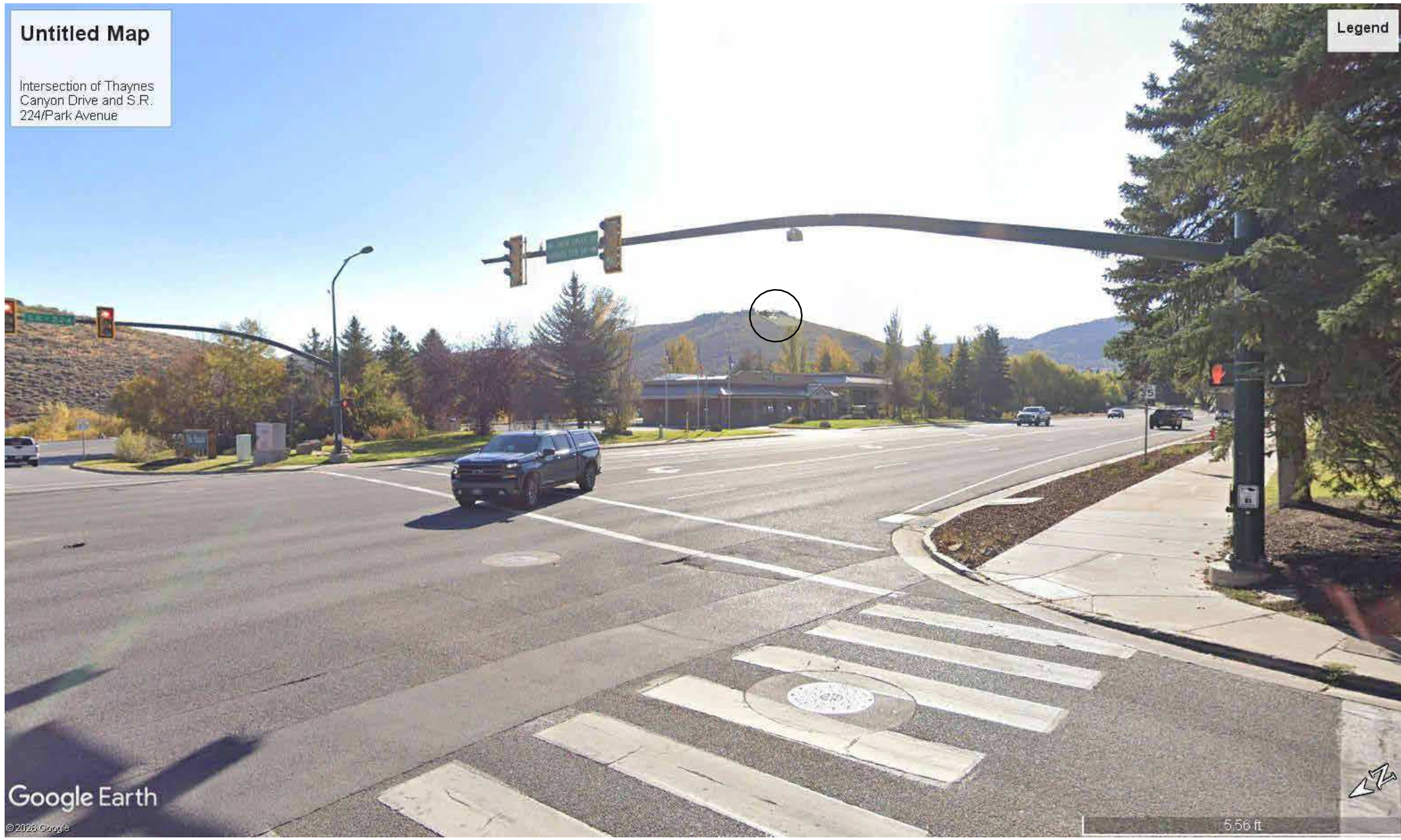
INTERSECTION OF THAYNES CANYON DRIVE AND S.R. 224/PARK AVENUE
