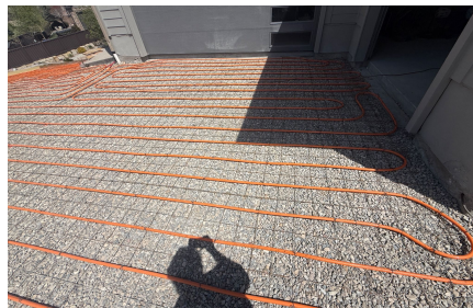
INSTALLATION PHOTOS - RADIANT TUBING PRIOR TO CONCRETE PLACEMENT
