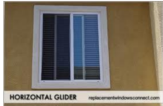
Not Allowed – Vinyl Windows
