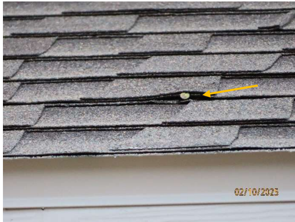
Exposed nail through a shingle at the center eave of the S/W corner south sloping roof covering
