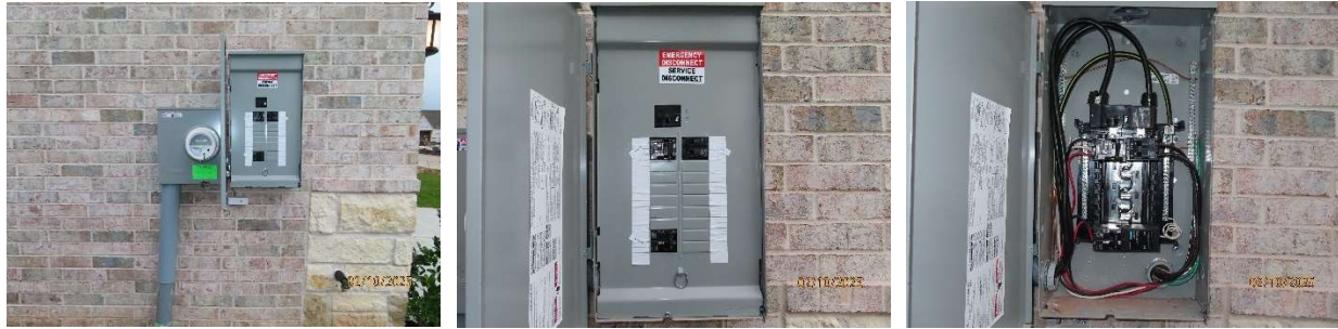
General views of the electrical service entrance lateral disconnect and distribution panel
