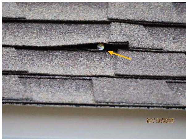
Nail lifting a shingle at the center eave of the south sloping roof covering
