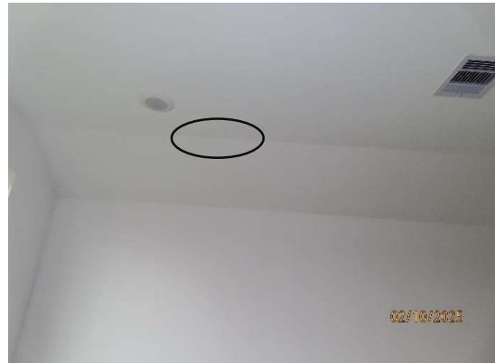
Drywall seam starting to separate at the east end center of the master bedroom south end vaulted ceiling
