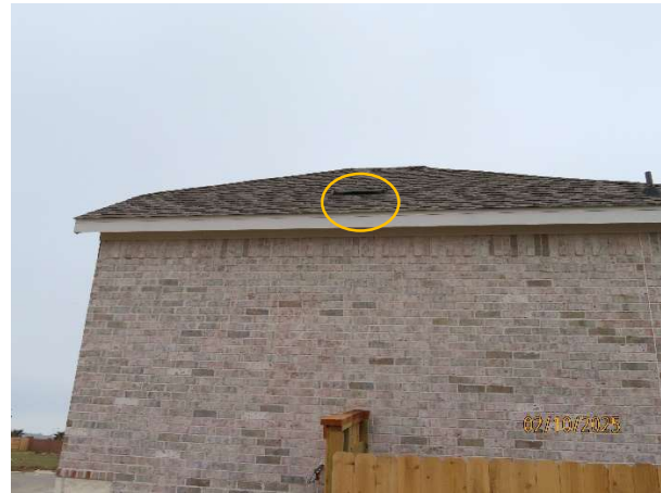
Exposed nail through a shingle at the center eave of the S/W corner south sloping roof covering
