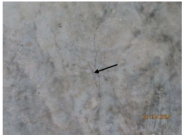
Examples of the closed hairline cracks through the center of the garage floor portion of the slab
