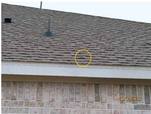
Nail lifting a shingle at the center eave of the south sloping roof covering
