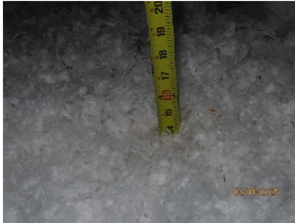
14 to 15 inches of loose fill fiberglass insulation on average
