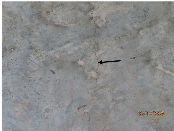
Examples of the closed hairline cracks through the center of the garage floor portion of the slab
