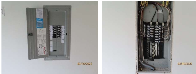
General views of the electrical service entrance lateral disconnect and distribution panel
