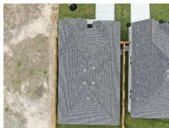
General views of the roof covering from above
