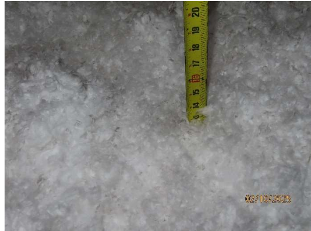
14 to 15 inches of loose fill fiberglass insulation on average
