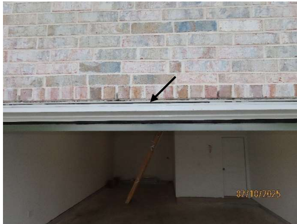
Gaps in between the header board and steel lintel plate along the top of the 16' garage door opening not reflective of significant settlement
