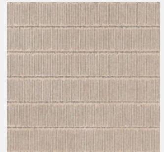
PORCELAIN COVERED ALL WALLS
