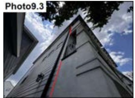
Siding & Stucco Termination / Seal
