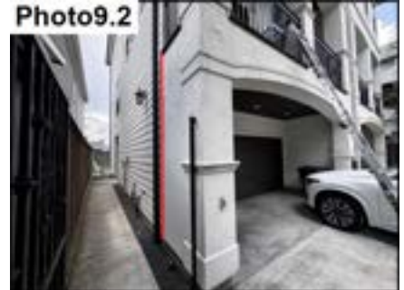
Siding & Stucco Termination / Seal
