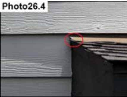
Roof Diverter Flashing Sealants / Seal
