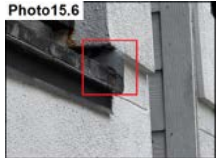
Balcony Flashing Sealants / Seal
