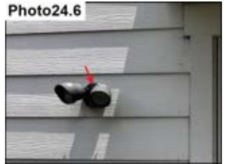
Penetration Sealants / Seal
