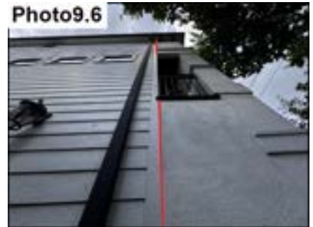
Siding & Stucco Termination / Seal
