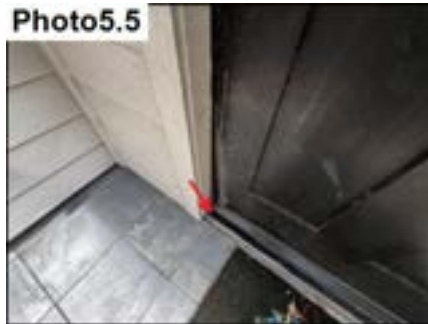
Door Trim and Miter Sealant / Seal
