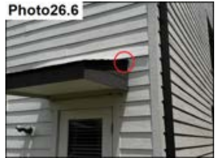
Roof Diverter Flashing Sealants / Seal
