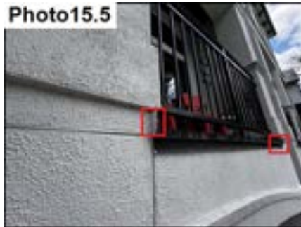
Balcony Flashing Sealants / Seal
