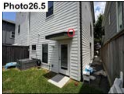
Roof Diverter Flashing Sealants / Seal
