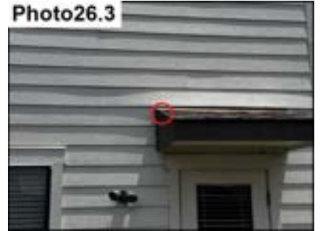
Roof Diverter Flashing Sealants / Seal
