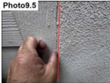
Siding & Stucco Termination / Seal
