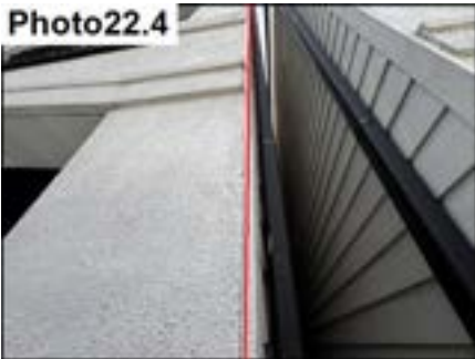
Siding & Stucco Termination / Seal
