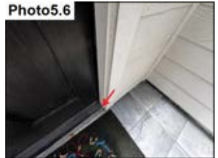
Door Trim and Miter Sealant / Seal
