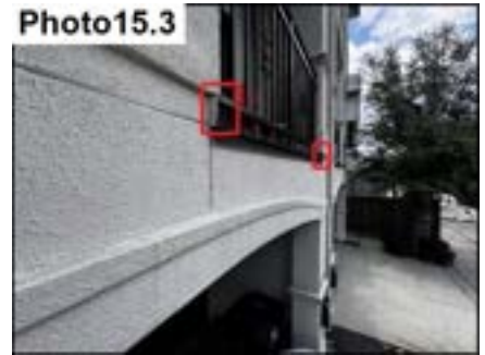
Balcony Flashing Sealants / Seal
