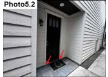
Door Trim and Miter Sealant / Seal
