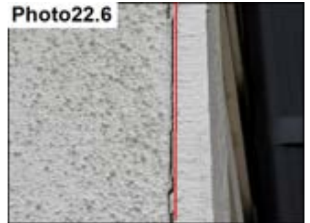
Siding & Stucco Termination / Seal
