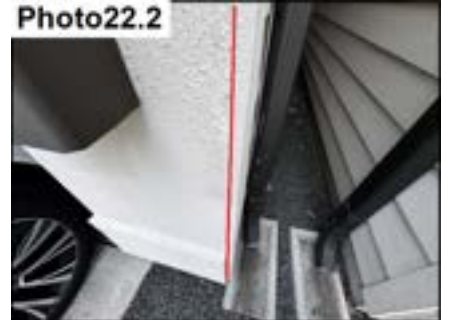
Siding & Stucco Termination / Seal
