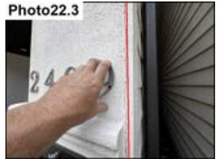
Siding & Stucco Termination / Seal
