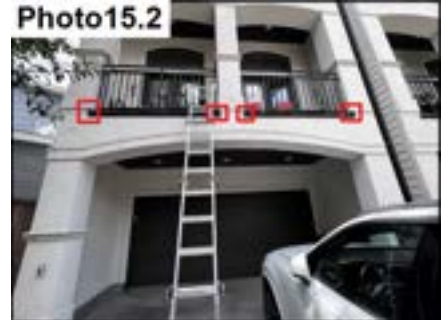
Balcony Flashing Sealants / Seal
