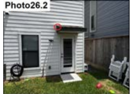
Roof Diverter Flashing Sealants / Seal
