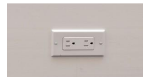
Outlets in baseboards
