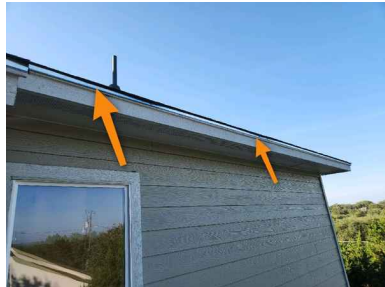
For Example: Unpainted Drip Edge Flashings
