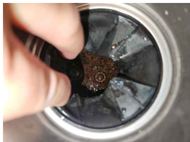
General Photos of Range Hood/Exhaust Systems:
