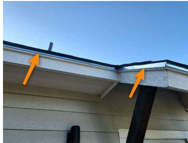
For Example: Unpainted Drip Edge Flashings
