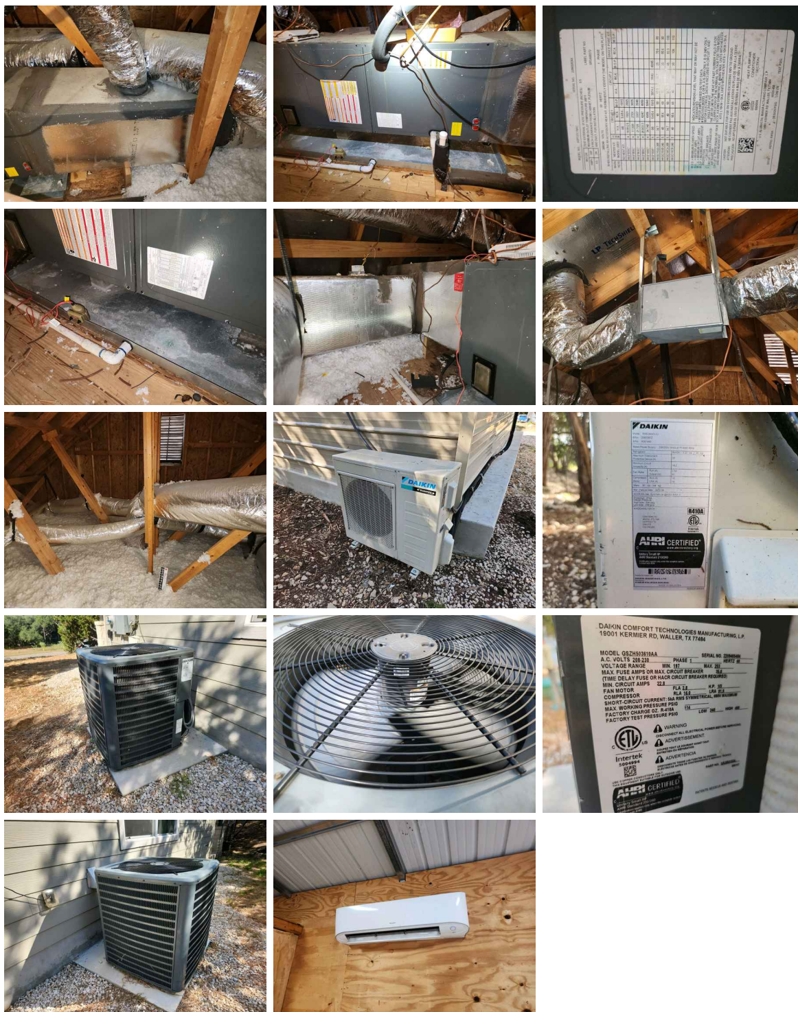
General Photos of Thermostats:
