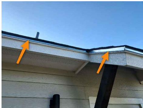
For Example: Unpainted Drip Edge Flashings
