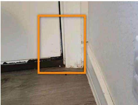
Visible Daylight at Side Entry
