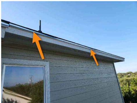
For Example: Unpainted Drip Edge Flashings
