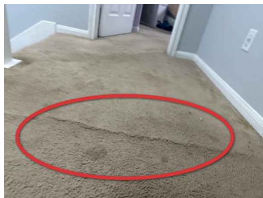
2nd Floor Hallway
