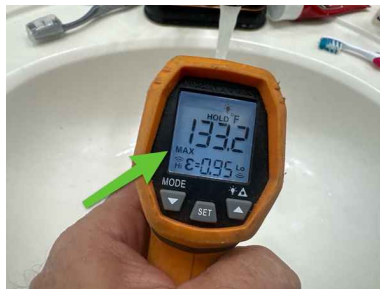
Hot water temperature
