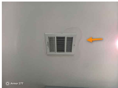
2nd Floor left bedroom
