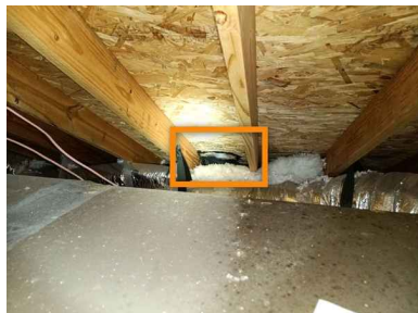
Middle of attic
