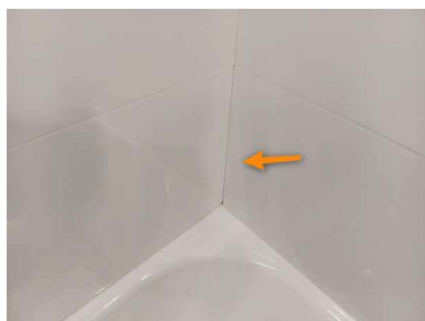
2nd Floor hall bathroom
