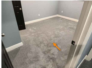
2nd Floor left bedroom
