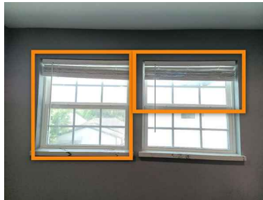
2nd Floor left bedroom
