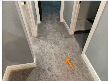
2nd Floor Hall
