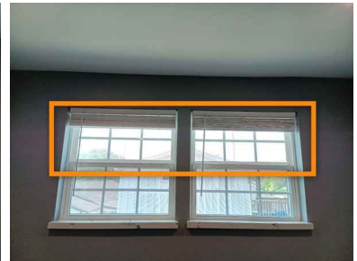
2nd Floor right bedroom
