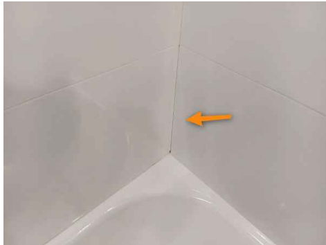
2nd Floor hall bathroom
