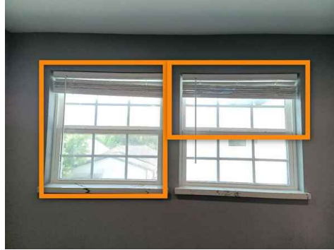
2nd Floor left bedroom
