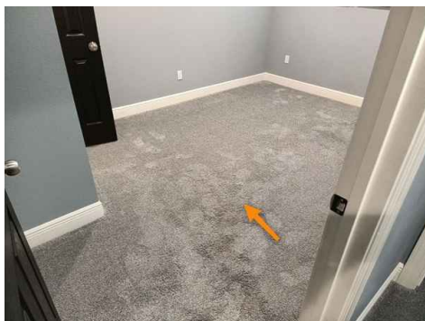
2nd Floor left bedroom
