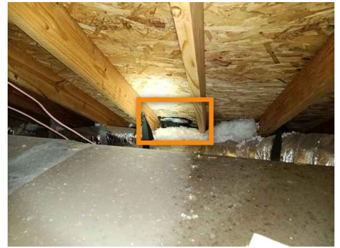
Middle of attic
