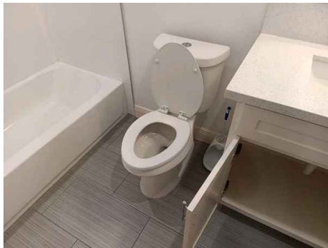
2nd Floor Hall Bathroom
