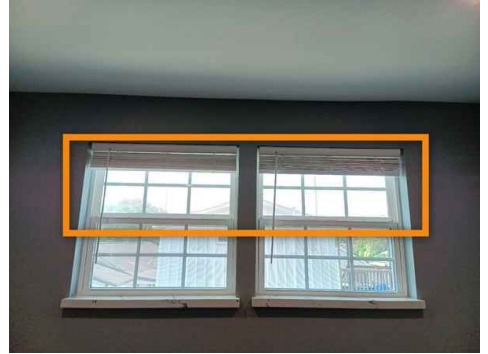
2nd Floor right bedroom
