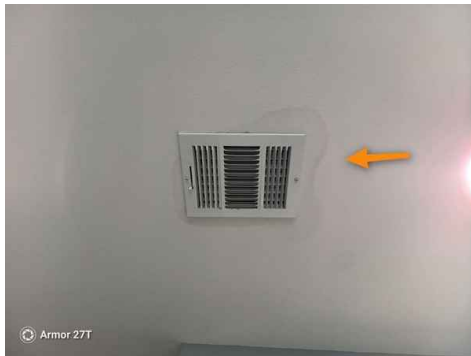
2nd Floor left bedroom
