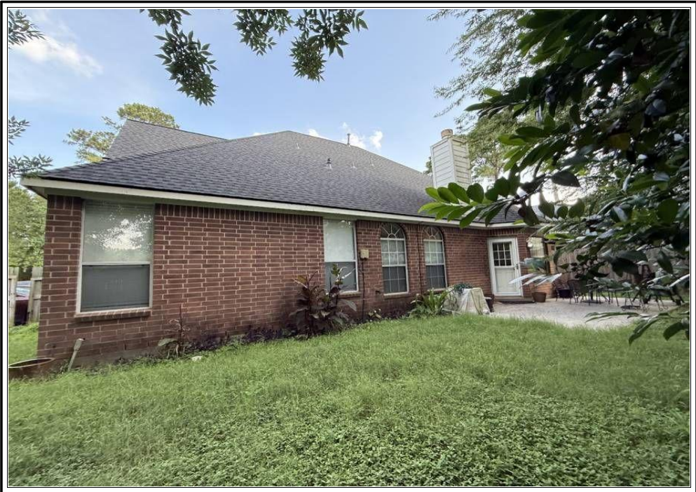
REAR OF SUBJECT PROPERTY
