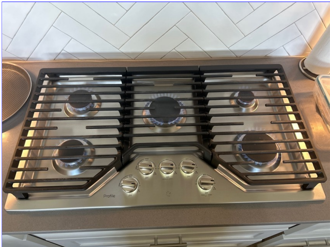
D. Item 3 (Picture) View of the gas range with burners lit for inspection
