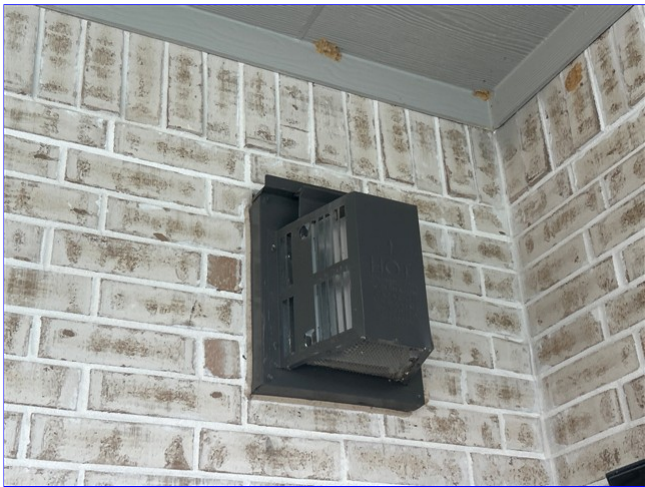
J. Item 2 (Picture) View of direct vent chimney
