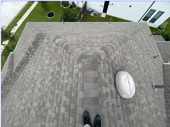
D. Item 4 (Picture) View of roof at the time of inspection
