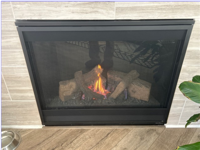
J. Item 1 (Picture) View of the fireplace lit for inspection
