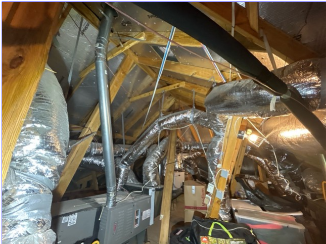
C. Item 1 (Picture) View of roof structure from attic space
