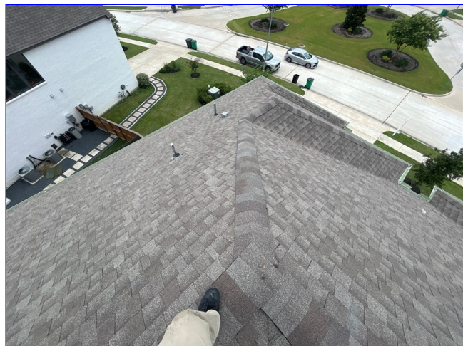
D. Item 3 (Picture) View of roof at the time of inspection
