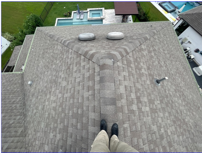
D. Item 5 (Picture) View of roof at the time of inspection
