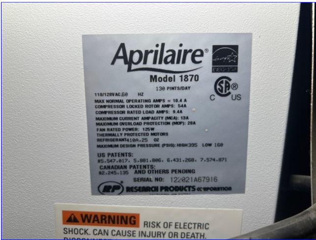
D. Item 3 (Picture) View of whole home dehumidifier data plate
