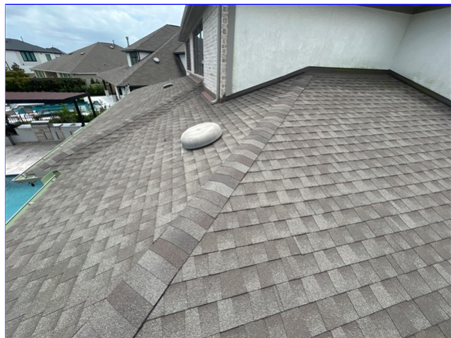
D. Item 2 (Picture) View of roof at the time of inspection
