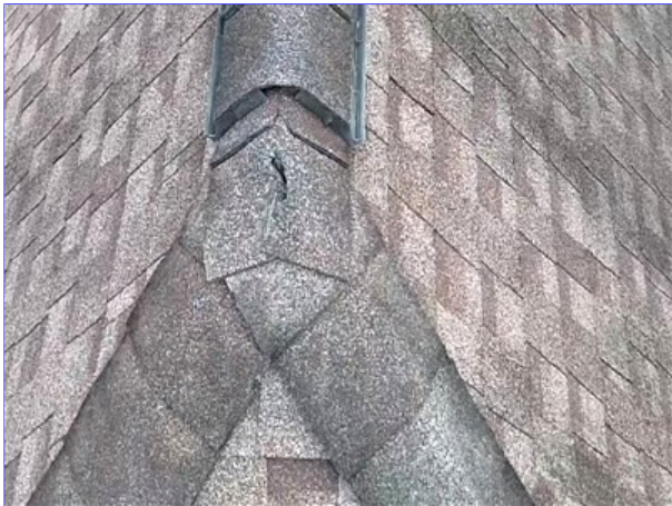
(4) Previous roof repairs were observed.
