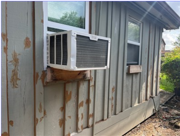
Garage apartment back
