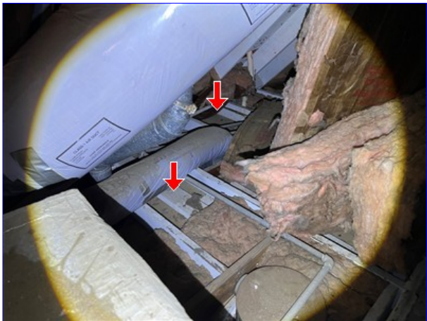
Ceiling attic access
