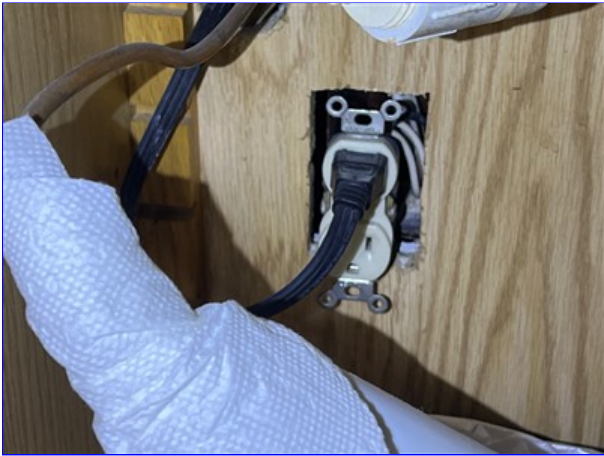
Kitchen wet bar cabinet
