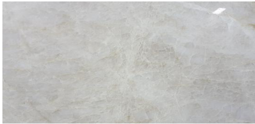
Bathroom Floor and Shower Walls
