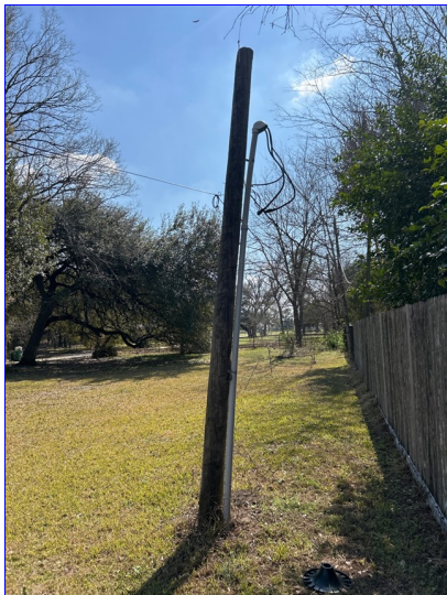
(6) The service pole is leaning. Recommend correction.
