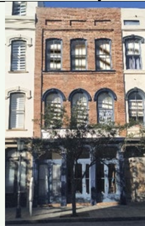
Tremont St. Facade
