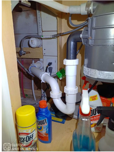
General Photos of Drain Lines:
