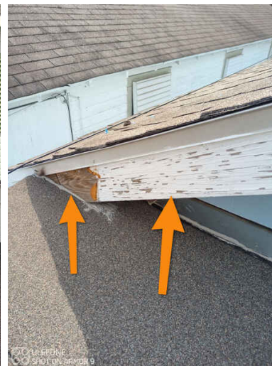
Rear of Front Roof
