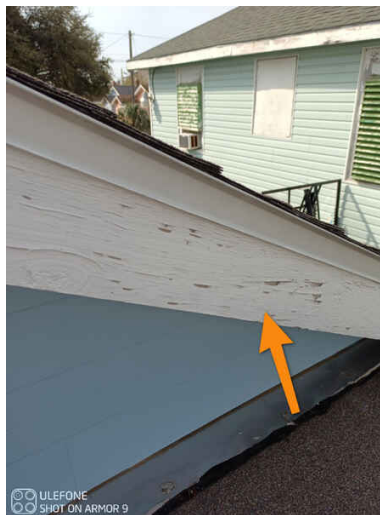
Rear of Front Roof.
