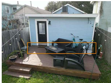
Rear of structure at Primary Bedroom
