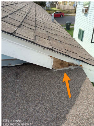
Rear of Front Roof
