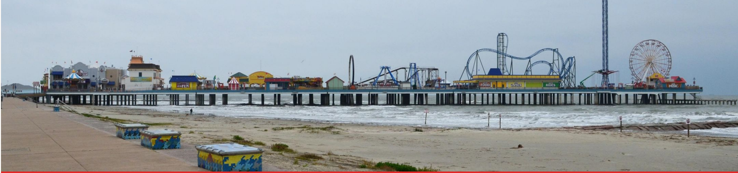
The Seawall and the Pleasure Pier
