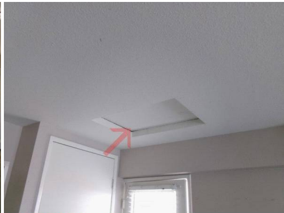
Garage attic access.
