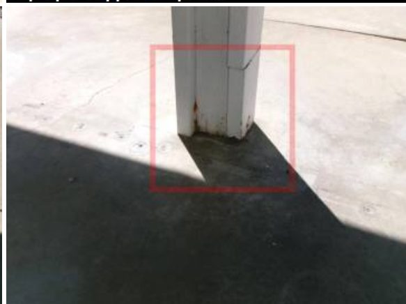
Improper support on posts.
