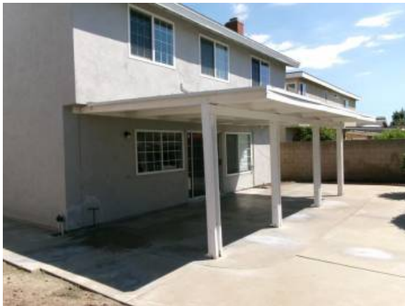
Improper support on posts.
