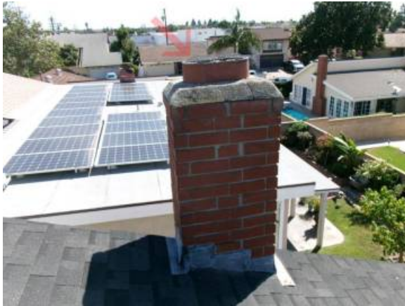
Cracks & damage to mortar cap.
