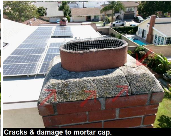
Cracks & damage to mortar cap.
