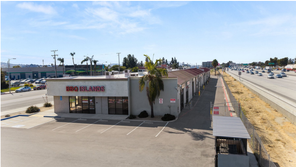
The building end, entrance and parking lot.
