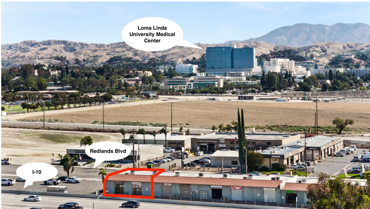
The units (outlined in red) along Redlands Blvd and I-10, with Loma Linda University Medical Center in the background.
