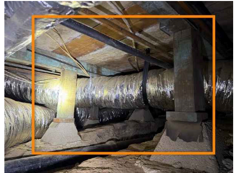
Various Locations Crawlspace
