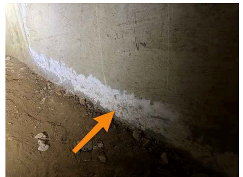
Rear Right Crawlspace
