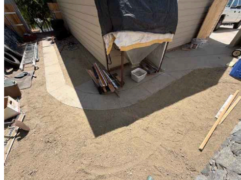
Garage Exterior Area
