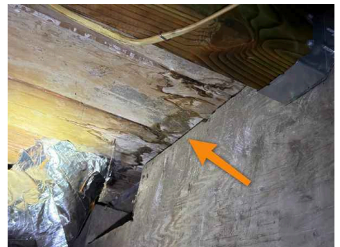
Rear Right Crawlspace
