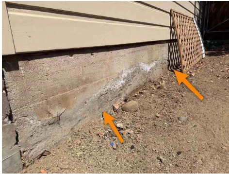
Right Garage Exterior
