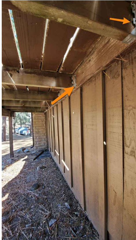
No fatteners of joists to hangers
