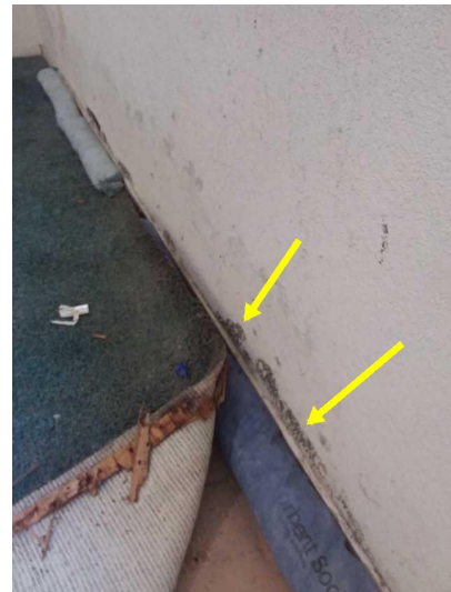
There is a mold-like substance that we will point out, which should be evaluated by a specialist. All molds flourish in a damp environment and many are commonplace, but some are toxic and represent a health threat.
