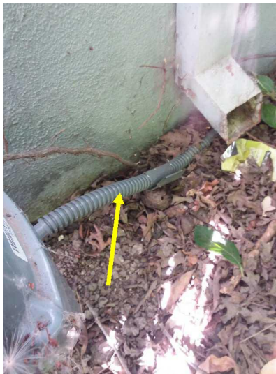
A gas pipe on the exterior of the home should be capped when not in use.
