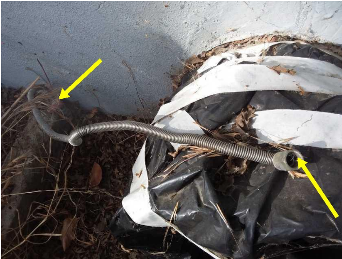
A gas pipe on the exterior of the home should be capped when not in use.
