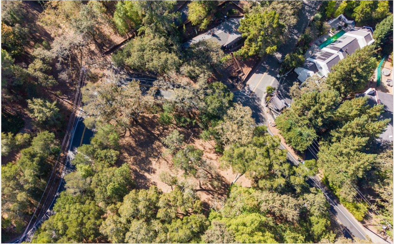
Overhead view of the site and Acalanes Road. Parcel lines are not drawn; see the locator in Section 4.
