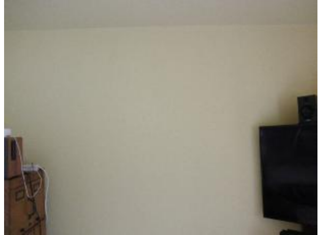
No water stains at the SW bedroom.
