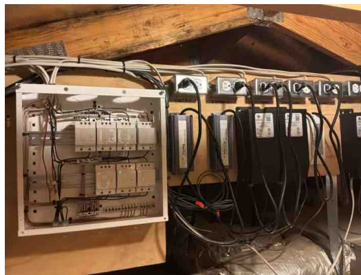
Example. Laundry attic
