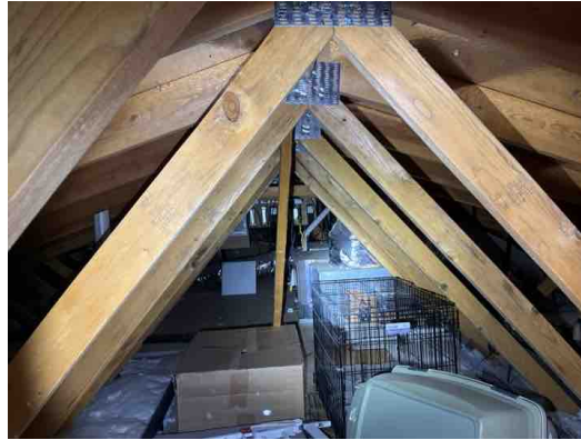
Example. Garage attic
