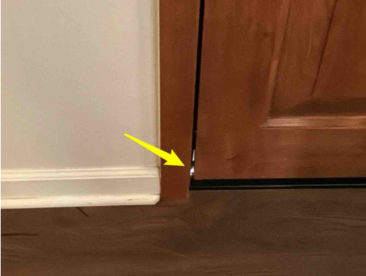
Laundry room hallway exterior door
