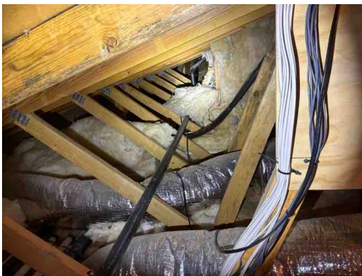
Example. Laundry attic
