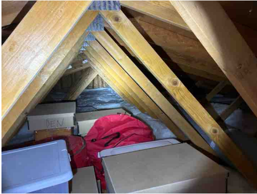
Example. Garage attic
