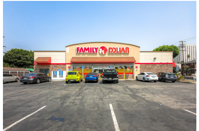
02 Front parking and storefront
